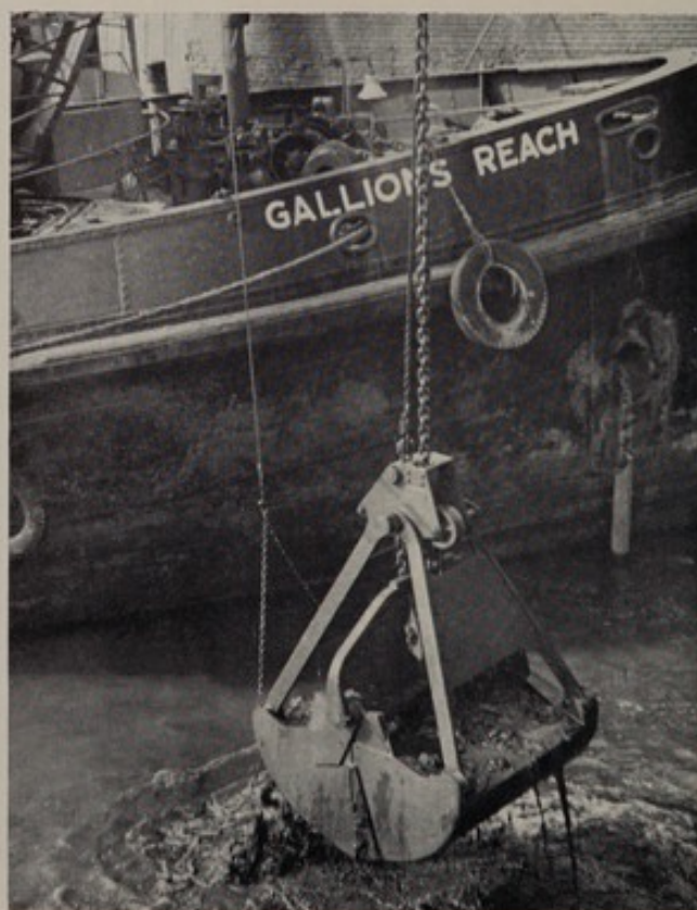
PLATE 12. Grab dredger working in Tilbury Tidal Basin
