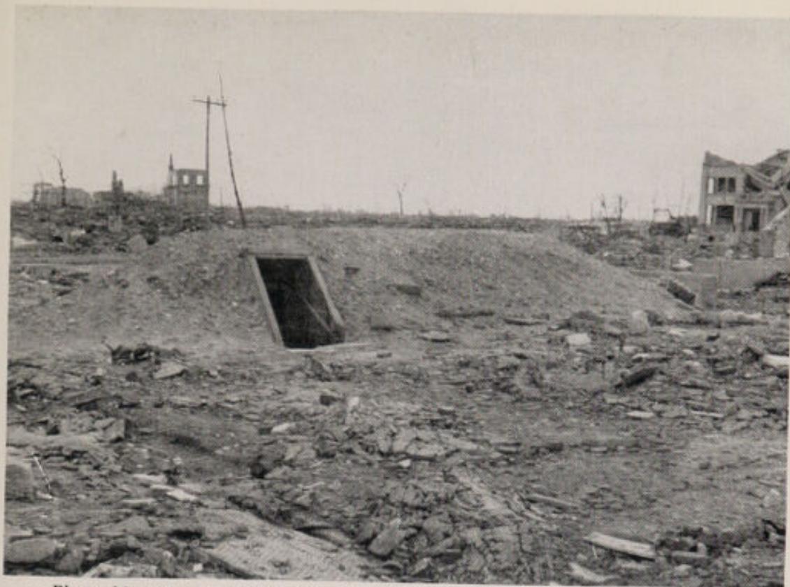
Photo No. 17. HIROSHIMA. Typical, part below ground, earth-covered, timber framed shelter 300 yds. from the centre of damage, which is to the right. In common with similar but fully sunk shelters, none appeared to have been structurally damaged by the blast. Exposed woodwork was liable to "flashburn." Internal blast probably threw the occupants about, and gamma rays may have caused casualties. See paragraph 40.
