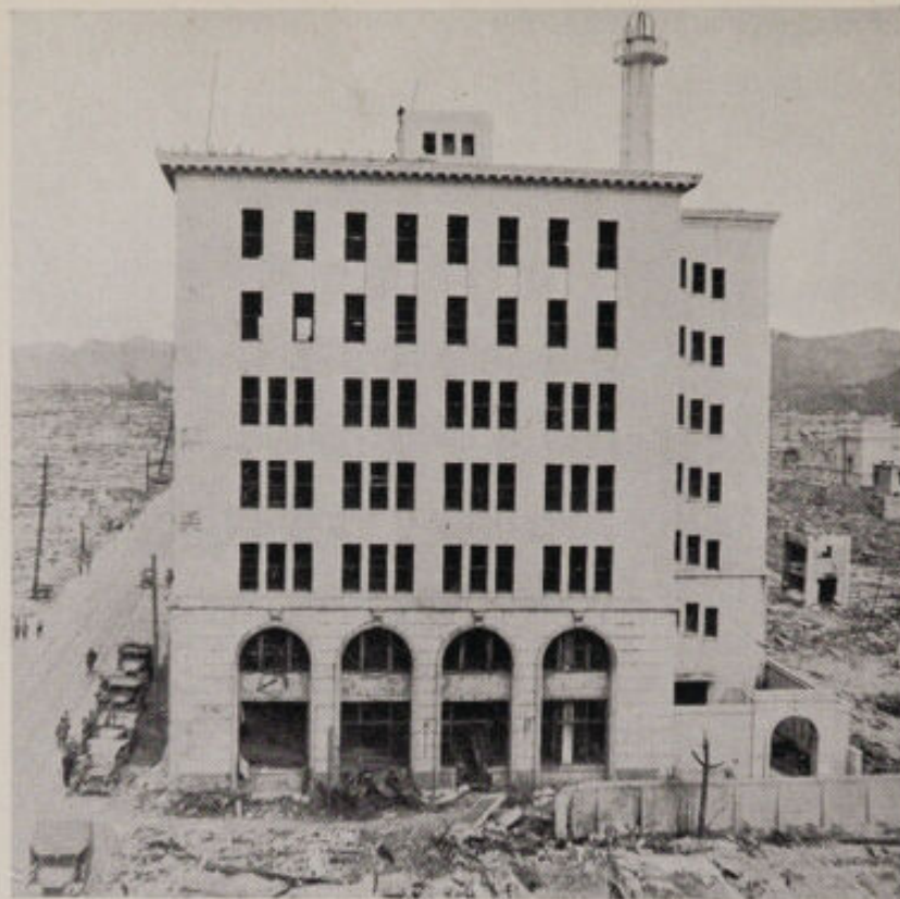
Photo No. 7. HIROSHIMA. Reinforced concrete building about 300 yds. from the centre of damage, which is to the left of the photograph. There was no serious structural damage, although a roof panel was depressed and some internal party walls were deflected. Designed for earthquake resistance, this building has a composite reinforced concrete and steel frame. See paragraph 24.
