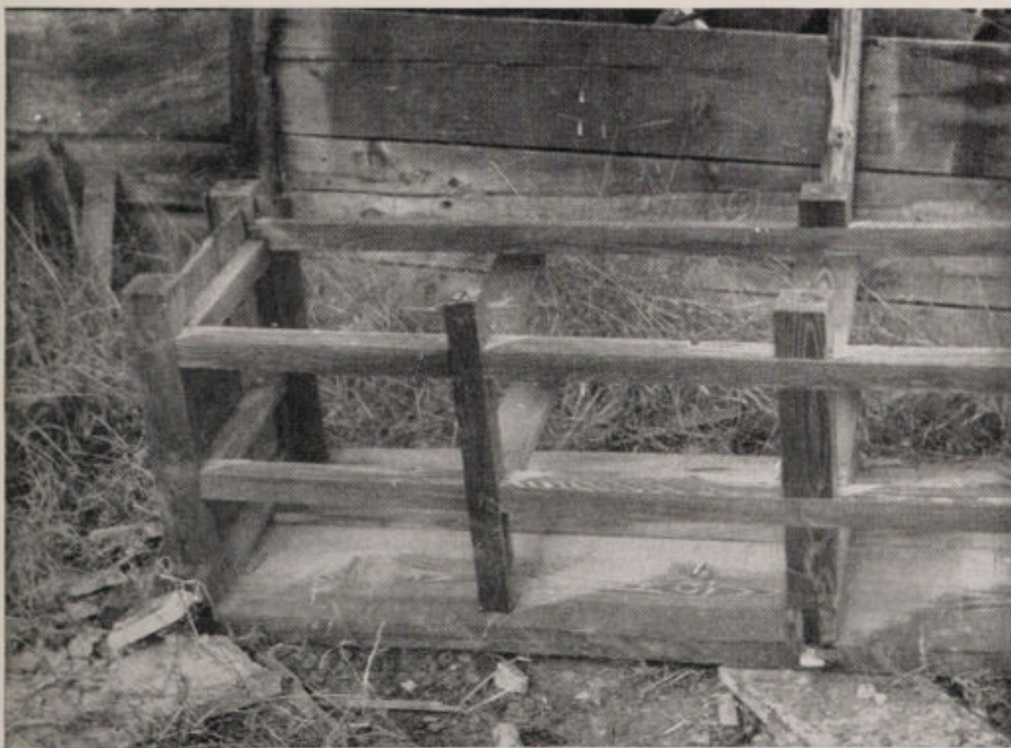
Photo No. 22. NAGASAKI. Timber framing scorched by heat radiation at \frac{1}{4} mile from the centre of damage. The surface is unscorched where it is shielded by the uprights. See paragraph 52.
