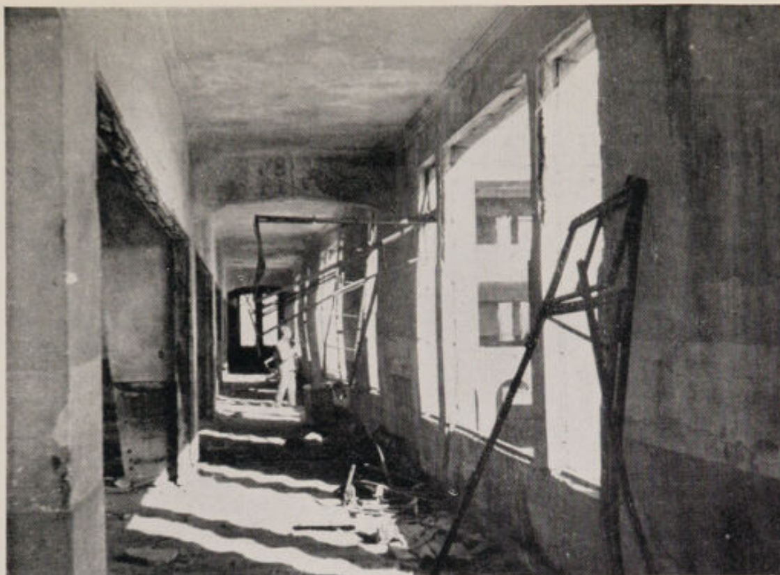
Photo No. 9. HIROSHIMA. Reinforced concrete school 500 yds. from the centre of damage, which is to the right. The frame of this building was of special design (portal) and resisted the lateral forces. The outside walls were of continuous reinforced concrete, and although they were deflected, as seen, they did not fail. See paragraph 27.
