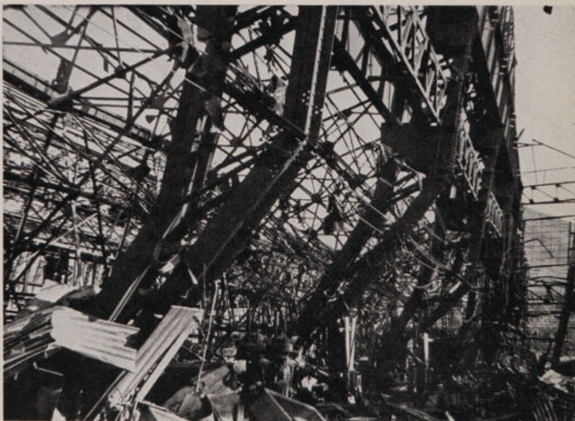
Photo No. 12. NAGASAKI. Large steel framed shed in the Mitsubishi Steel Works, \frac{1}{4} mile from the centre of damage. The steel stanchions have been bent (away from the explosion) and the roof trusses on both sides of these stanchions have collapsed. See paragraphs 22 and 32.
