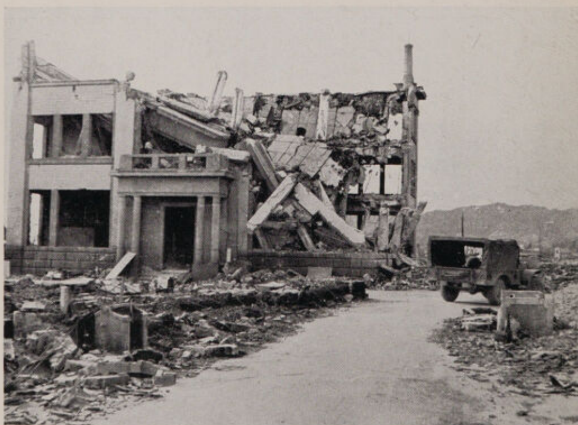
Photo No. 8. HIROSHIMA. Reinforced concrete building 200 yds. from the centre of damage, which is to the right. The blast from the bomb forced the roof slab down, the slab shearing round the column heads, leaving the internal columns projecting through the debris. Few concrete buildings failed in this way. See paragraph 24.
