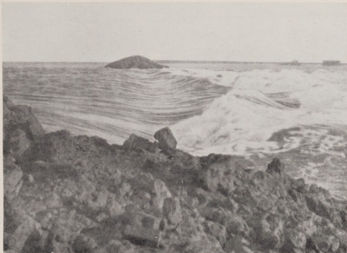
Plate 17. Rupture of a dyke (1916) ; sea pouring into the Anna Paulownapolder. This polder, one of the largest in the Netherlands, lies in the extreme north of North Holland. It was drained in 1847.
