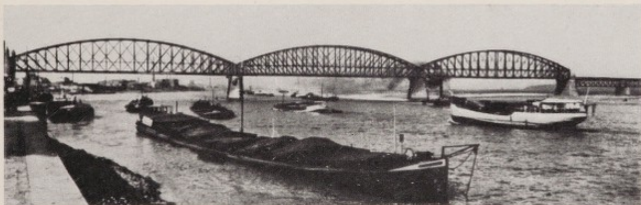
Plate 99. Maastricht : Wilhelmina bridge (R. Maas), looking downstream The town lies on the left bank. The bridge was opened in 1932 ; upstream is the thirteenth century St. Servais bridge ( Oude Maasbrug ), reconstructed in 1932-3. Each bridge has, on the east side, a wide and high span to facilitate navigation. On the left bank is the lateral canal joining the Zuid-Willemsvaart and the Maas-tricht-Liège canal.
