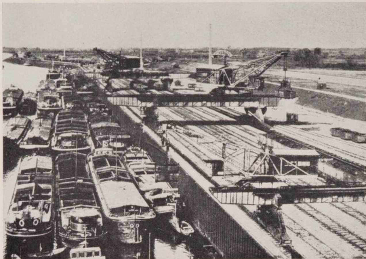
Plate 88. Juliana Canal : the coal port of Stein, looking north The three transporters each have a capacity of 20 tons.
