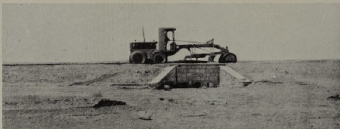
141. Auto-patrol laying the surface mat over a desert culvert
