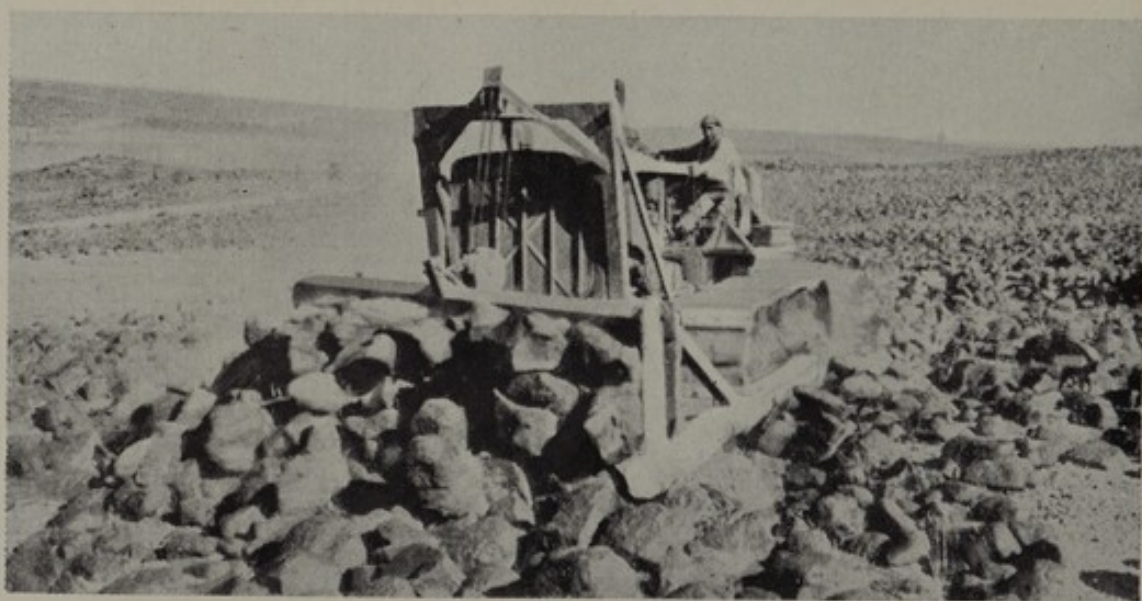
142. Motor-mechanical angle-dozer clearing a track in the lava belt
