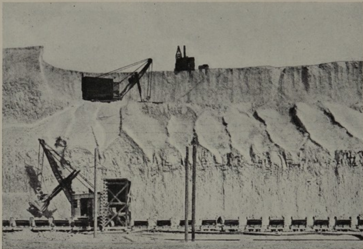
Plate 56. Limestone quarry in north-east Jylland (Jutland) The limestone is used, with clay, in the manufacture of cement.
