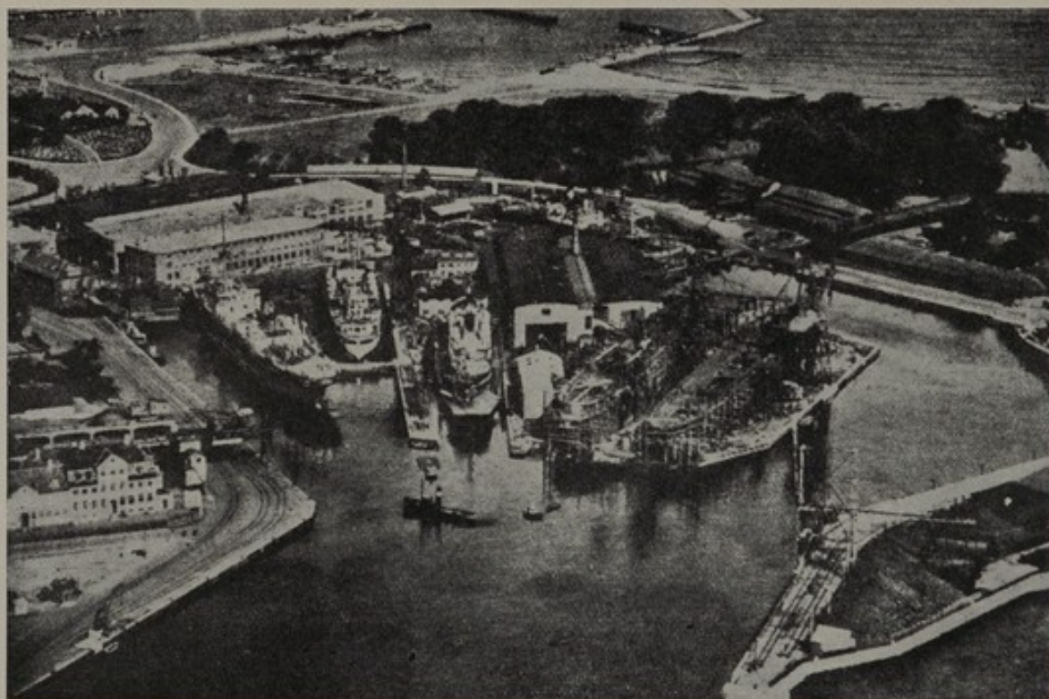
Plate 53. The shipbuilding yard and engineering works at Helsingör (Elsinore) The view is taken looking north from the entrance to the harbour. On the right are the two building slips. To the left of these is a ship on the patent slip, another is in the dry dock, and a third is moored alongside the east quay of Vestre Havn (cf. plan facing p. 436). A part of the fishing and yacht harbour (Helsingör Nordhavn), which lies north of Kronborg point, can be seen in the background.
