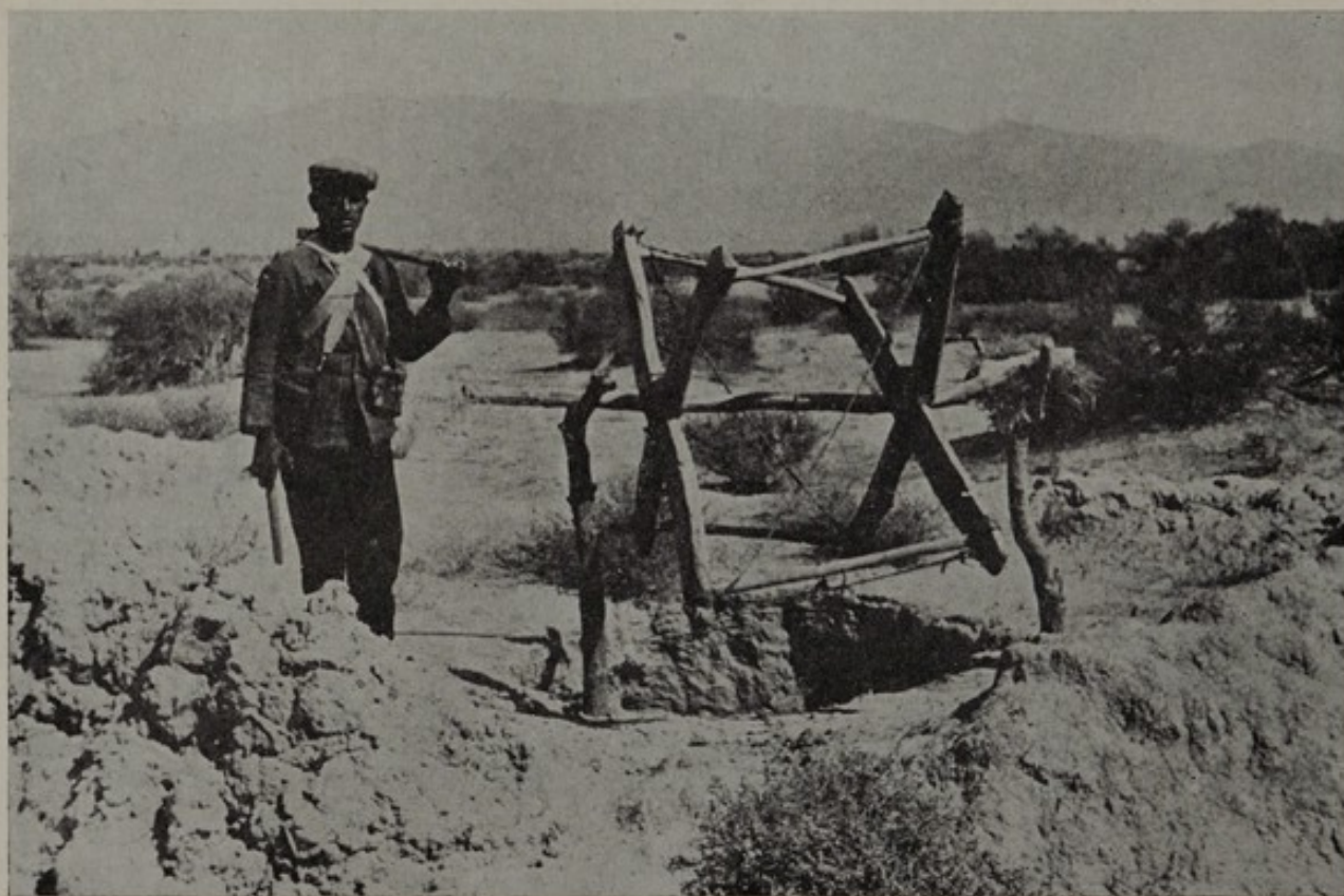
229. Windlass and shaft for excavating a qanat
