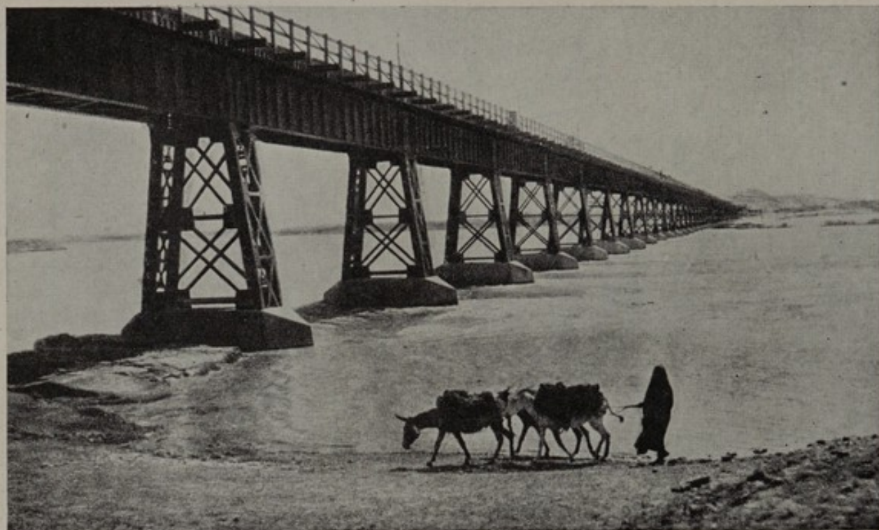
321. Bandar Shāhpur–Tehran railway. Steel bridge, 1,165 yards long, over the Karun river at Ahwāz
