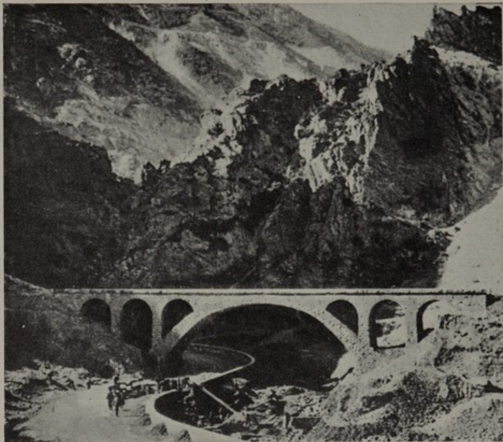
331. Bandar Shah-Tehran railway. Motor-road passing under railway bridge (span 82.5 feet) near Vresk station
