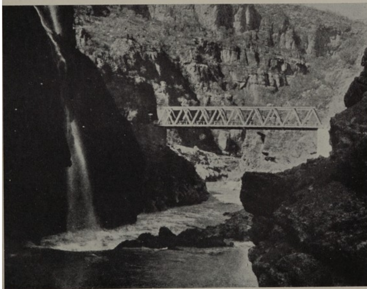
227. Single Hopkins-span bridge, 45 yards long, over the Ruwandiz river in the gorge below Ruwandiz, 65 miles from Erbil
