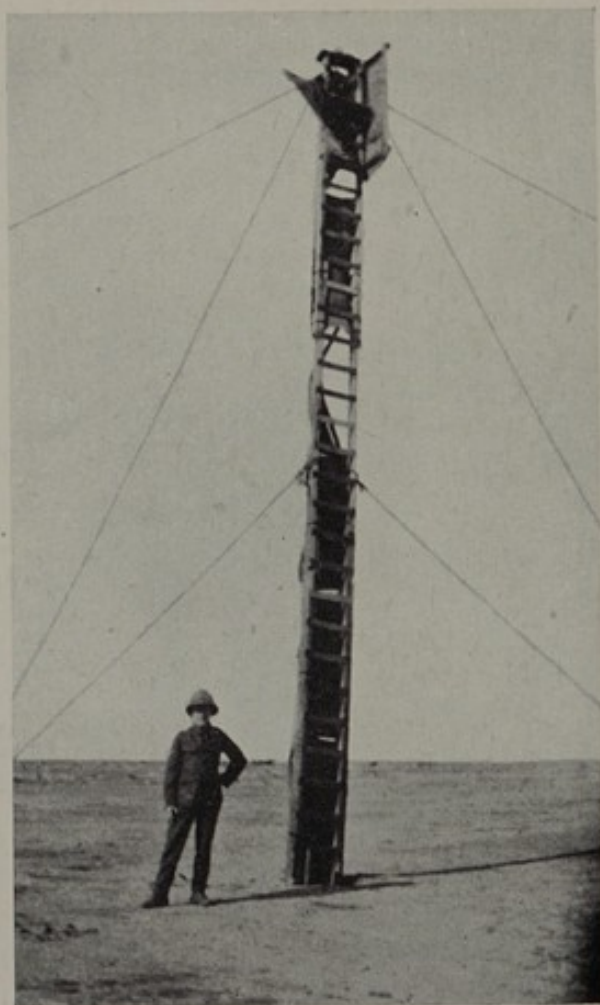
73, 74. Mirage. Types of artillery observation ladders rendered necessary by mirage
