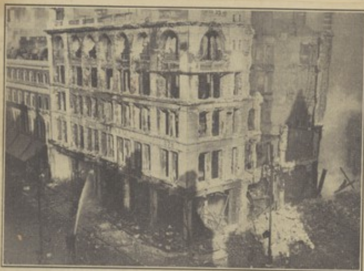
BIG STORE FIRE.—Several stores in Oxford Street were hit during Tuesday night's raid. Above is that of Lewis's, which suffered heavy damage. 17-9-41
