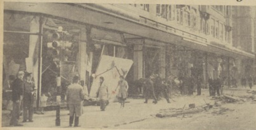
Debris from shattered windows littering the pavement outside a West End store to-day. Girl workers are helping A.R.P. squads to clear up. George Halliday
