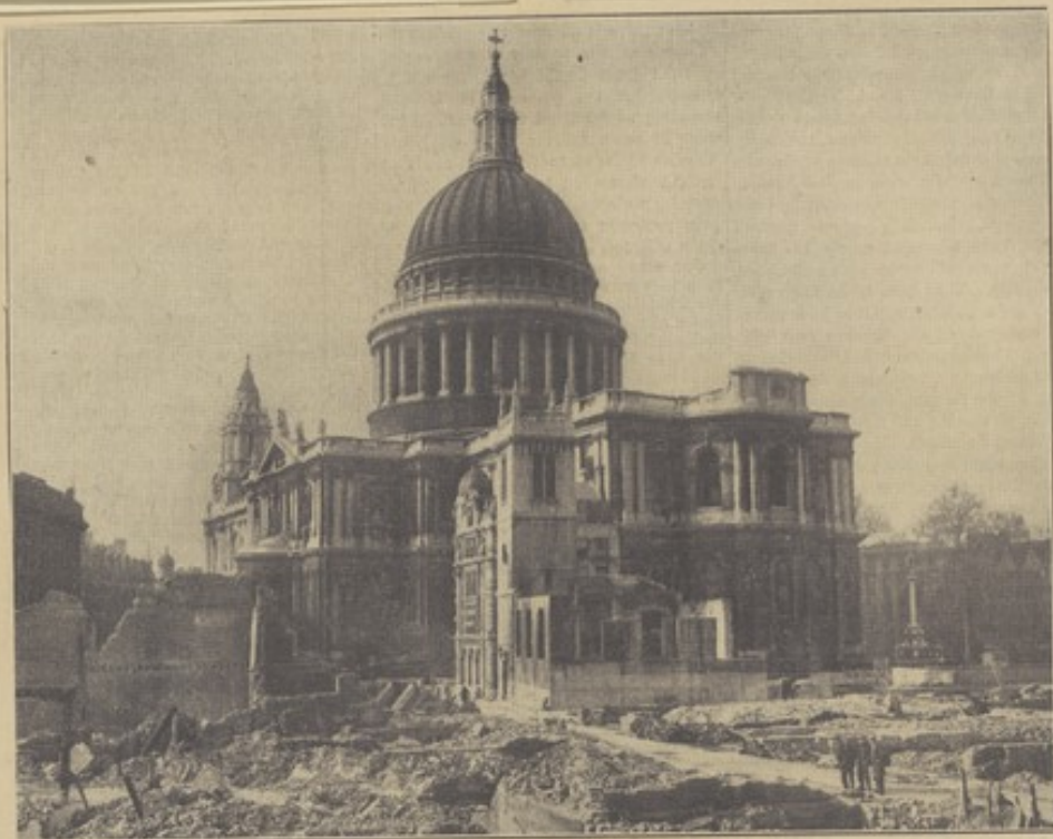
ST. PAUL'S CATHEDRAL as it can now be seen from the south side of Watling Street. Now that the remains of many demolished buildings have been cleared away the grandeur of Wren's conception from the east side is revealed for the first time to modern eyes. The tower of the little church of St. Augustine, rebuilt by Wren in 1683, now takes its place "in the picture," and the Cross in the churchyard is also for the first time visible from the same viewpoint. Time 26.2.42
