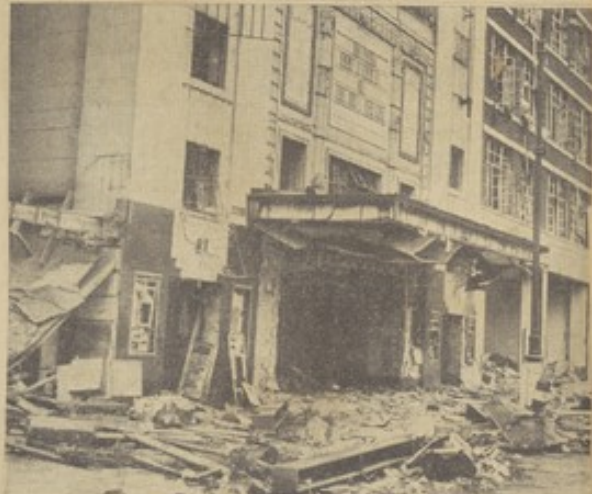
Bomb damage to a cinema in the Central London area—to-day's W. of St. P. Tamworth picture. Night of 18-9-40
