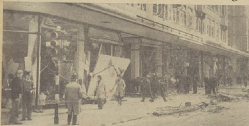
Debris from shattered windows littering the pavement outside a West End store to-day. Girl workers are helping A.R.P. squads to clear up. Comma Hallgruud
