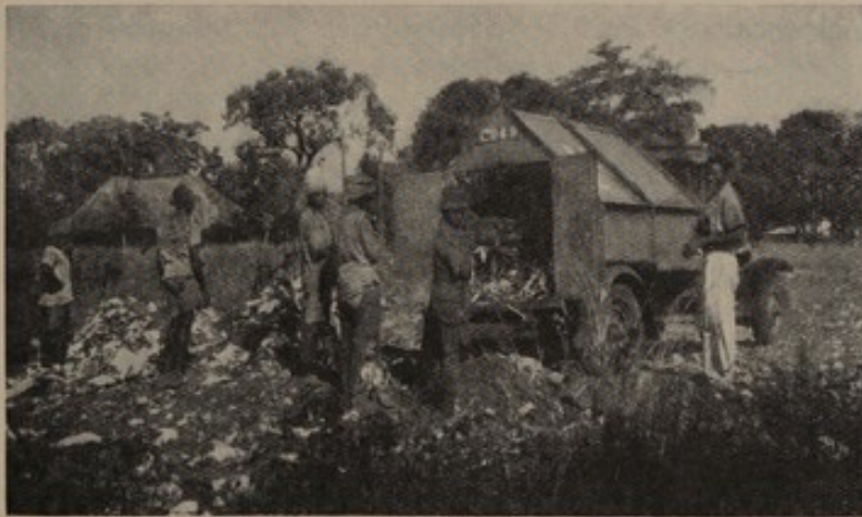
Dumping Refuse in old disused Pits.
