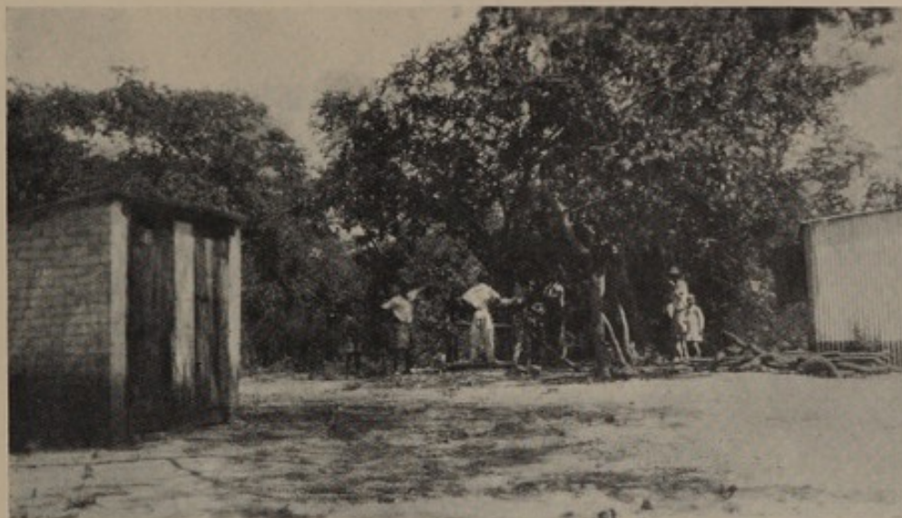
Shallow well providing water for European household. Note the absence of a protecting wall to well and the proximity of pit latrine.
