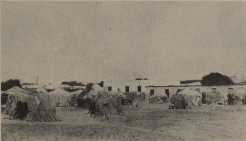
1931. Housing for Railway Employees at Ndola.
