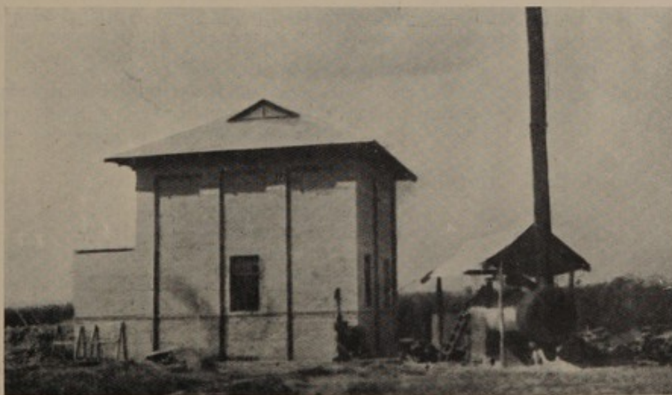
New Borehole and Pumping Station.
