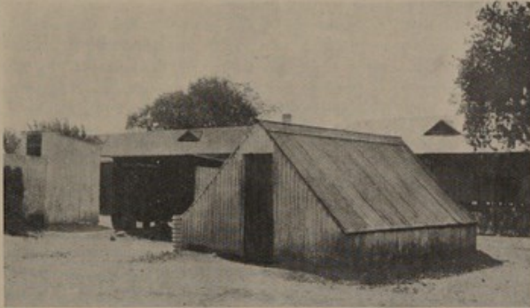
Personal Servants' Quarters built of galvanised iron with walls of 1 ft. to 1 ft. 6 ins.
