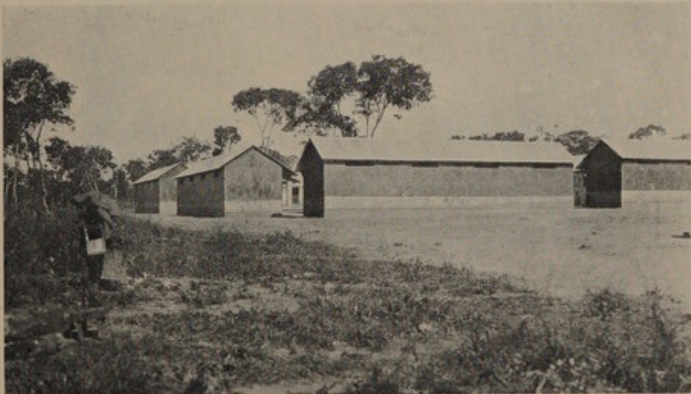
Back view of same.
