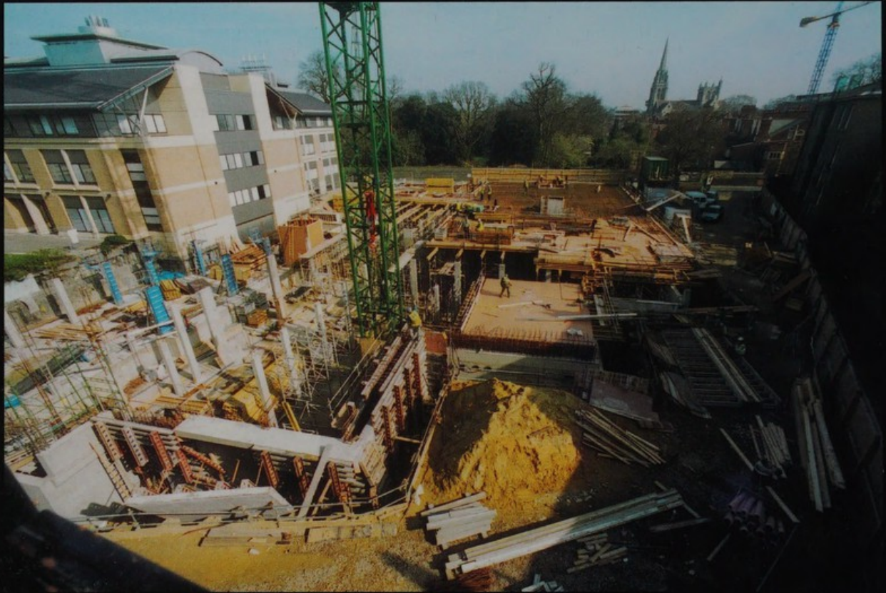
Our new building under construction
