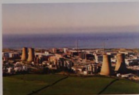
British Nuclear Group Reprocessing plant (THORP) at Sellafield
