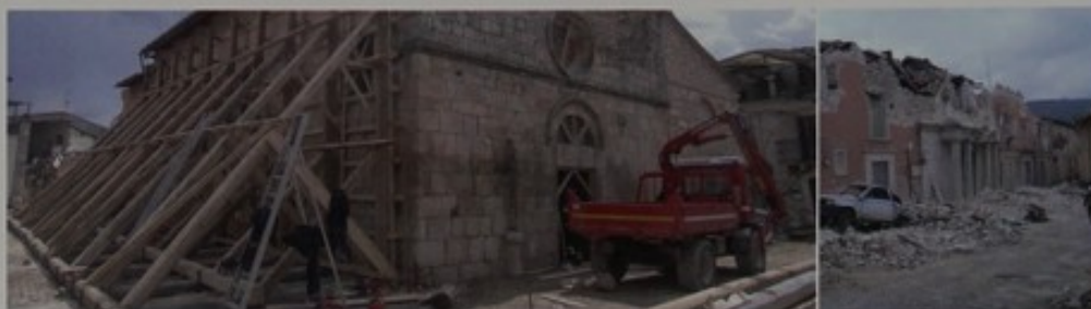
Left: Propping up the San Paolo Apostolo Church in Onna; right: Damage to the Prefecture building in L'Aquila.
