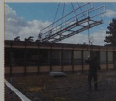
Fire protection at JRC-ITU: Installation of a new emergency evacuation bridge for the administration building
