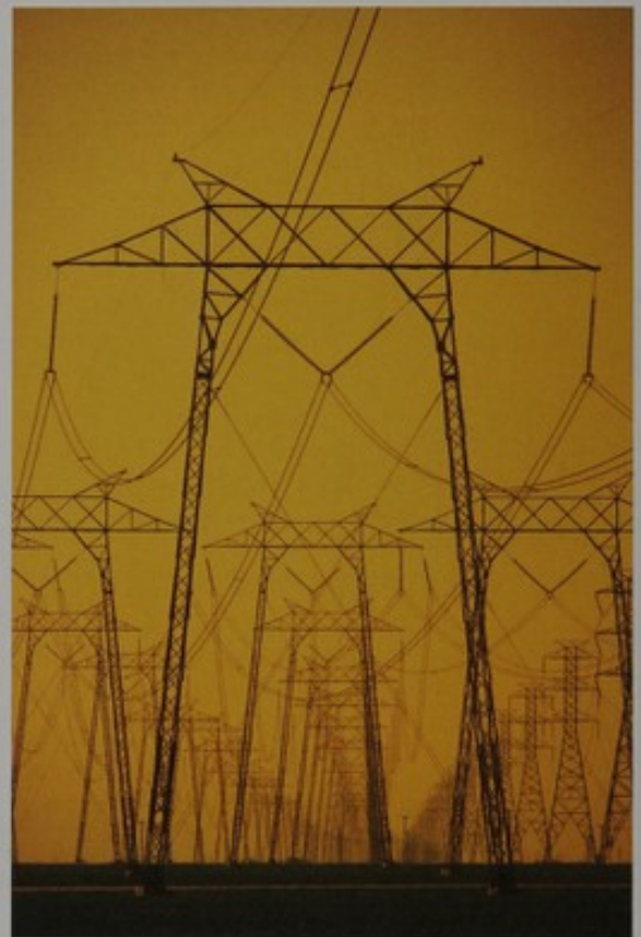
Electricity pylons in the sunset
