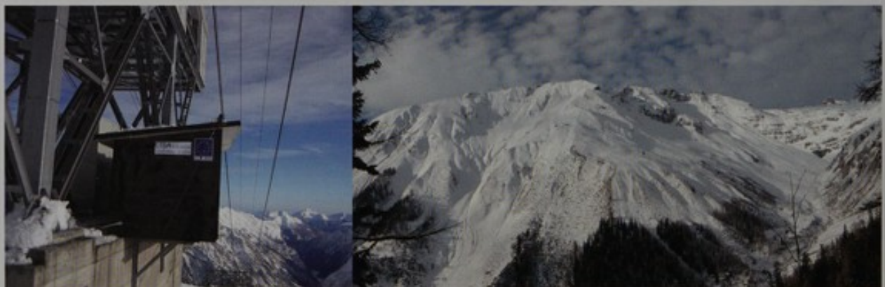
Monitoring Avalanches in Alagna, Italy
