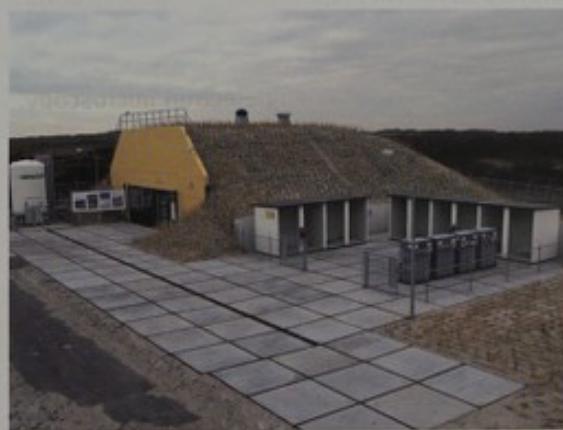
The H 2 tank testing facility
