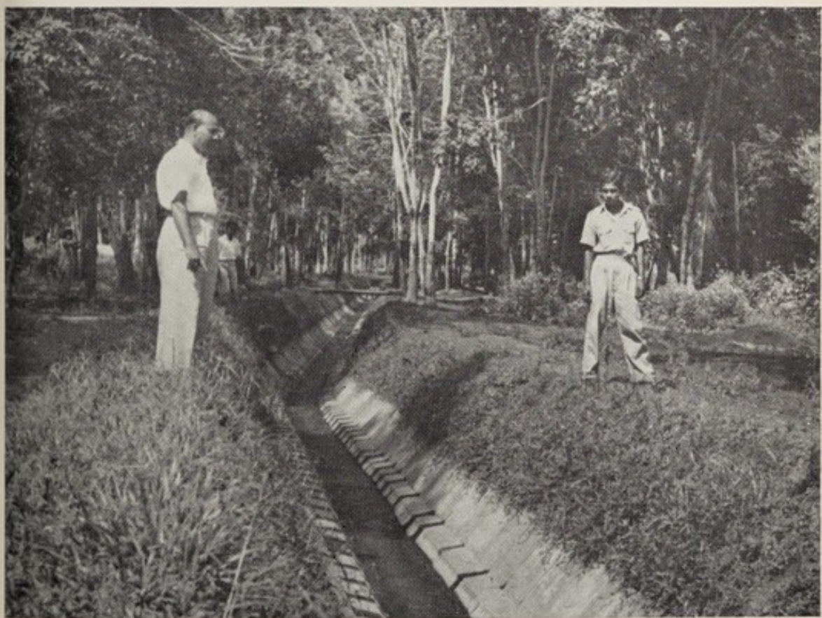
Completed portion of Channel Drain showing storm water ledges and storm water discharge pipe
