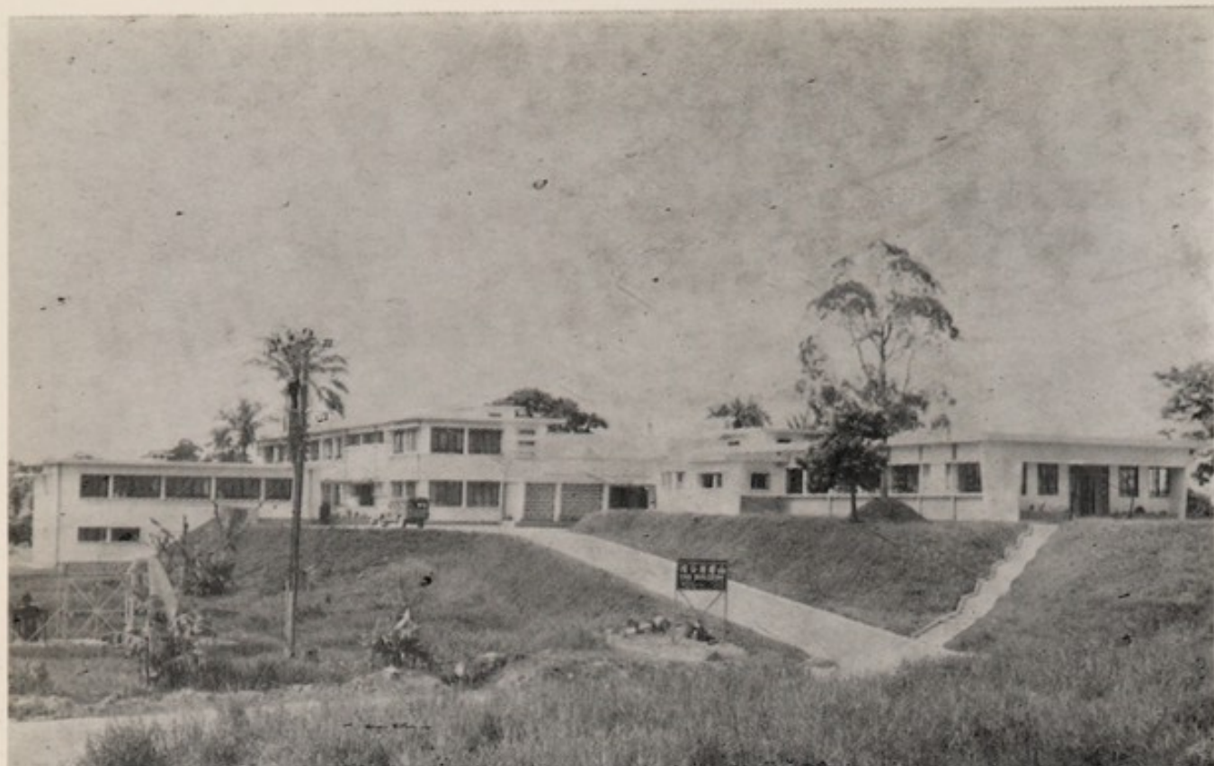
The New Simanggang General Hospital
