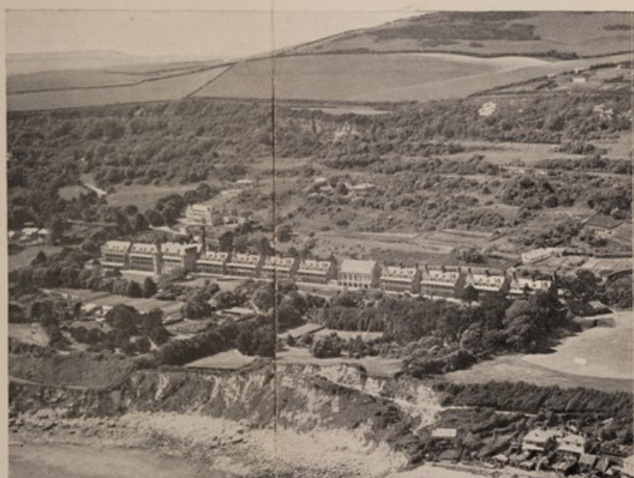
Aerial view showing Grounds, and Downs forming protection from North.
