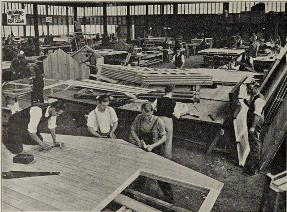
THE PORTABLE BUILDINGS DEPARTMENT
