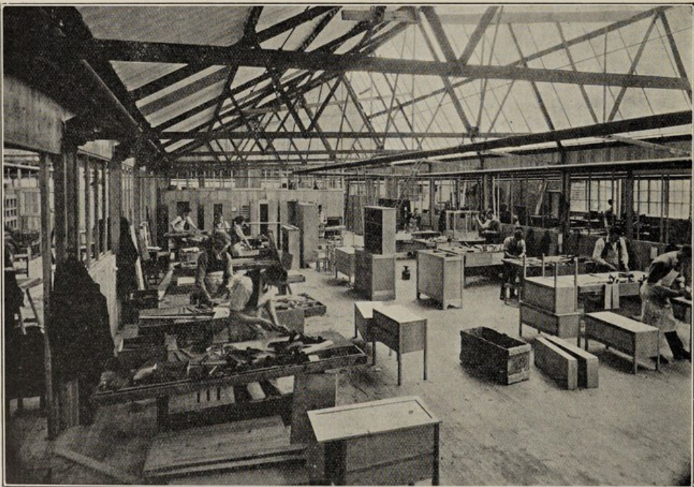
ANOTHER VIEW OF THE MAKING SHOP
