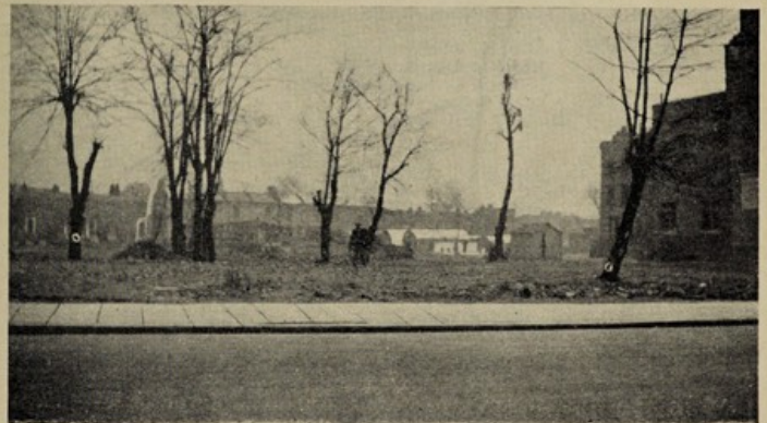
View from the Annie McCall looking across Jeffrey's Road, giving an idea of the extent of the damage in its vicinity. Temporary houses are being erected here
