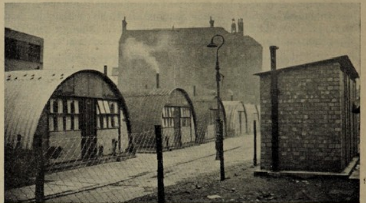
Temporary houses on the large site adjoining Mildmay Mission Hospital, some of them on hospital property. The hospital is in the background
