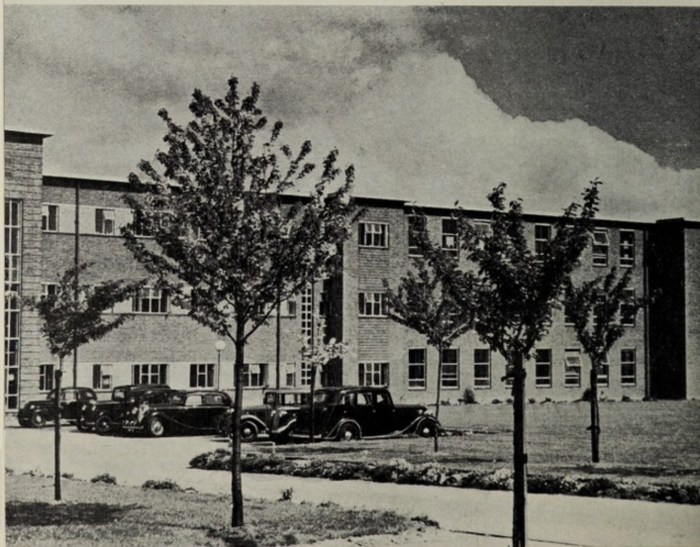
Ward Block seen from the Main Entrance
