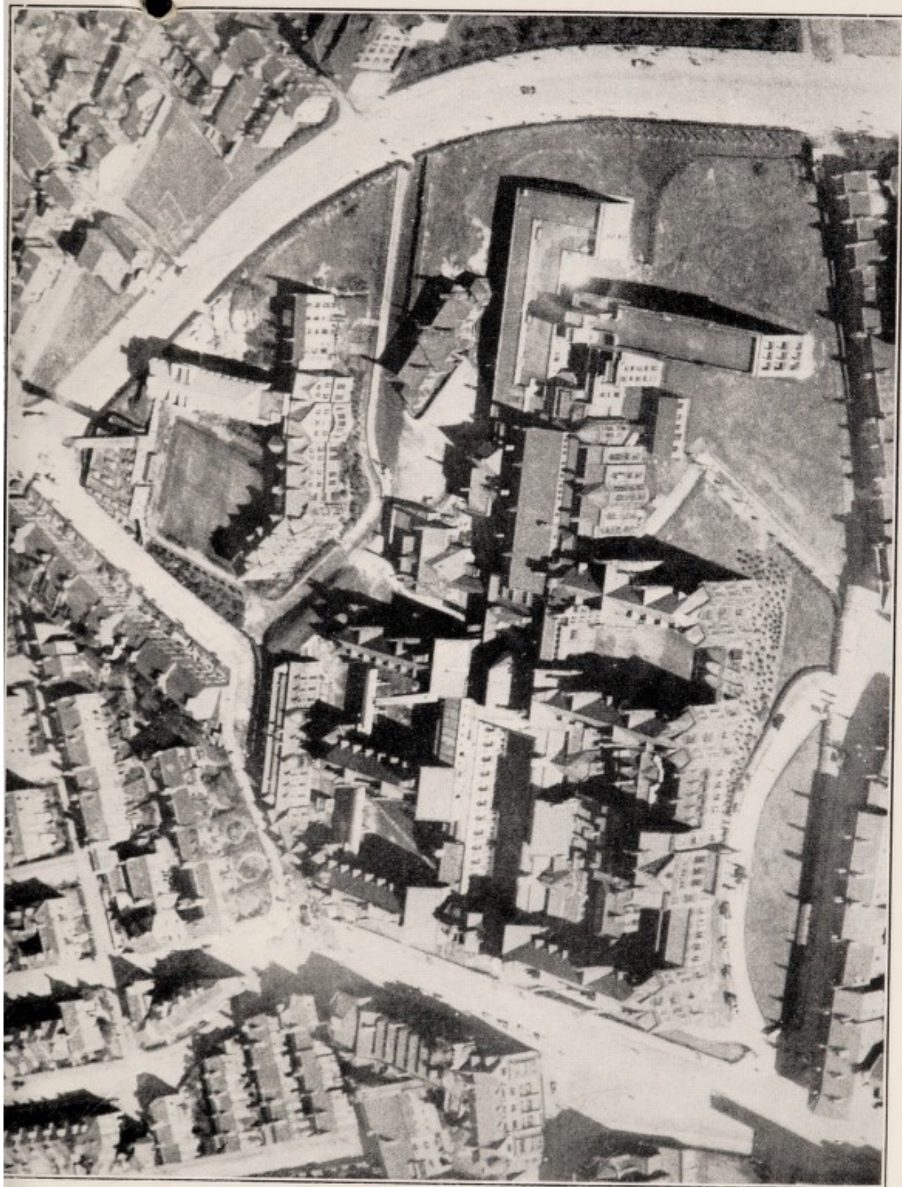
AERIAL VIEW OF THE INFIRMARY.
