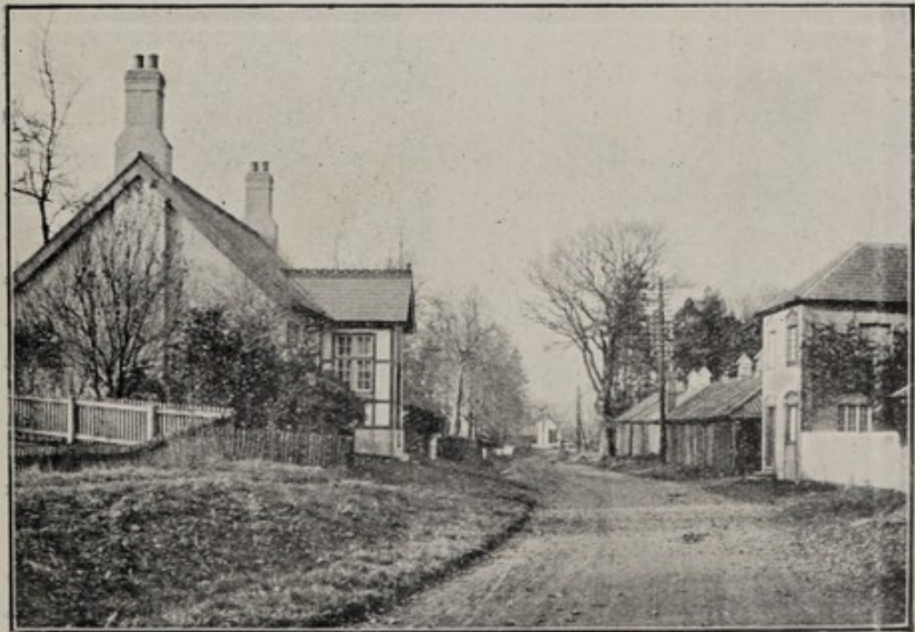
ESTATE OFFICE, ERMINE STREET.
