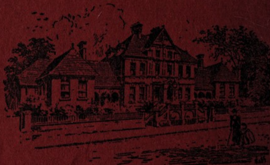
FRONT VIEW, NORTH STREET.
