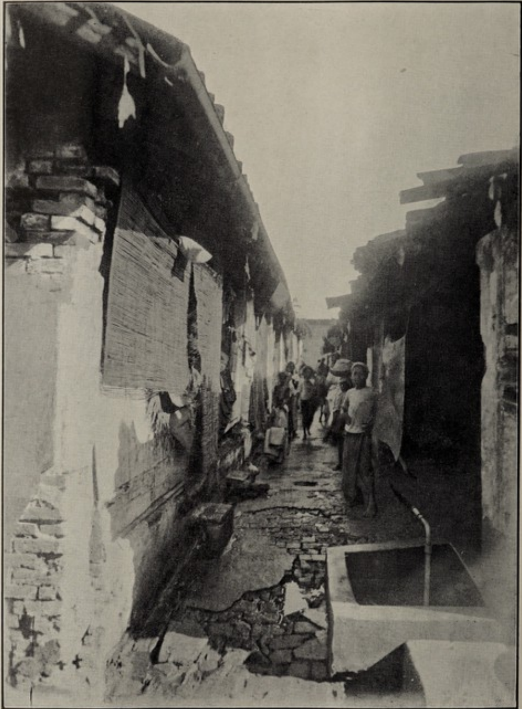
4/4 B, VINCENT STREET, BEFORE IMPROVEMENT.
