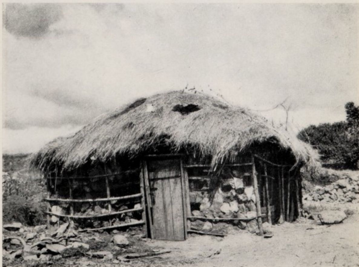
Problems still to be tackled—typical peri-urban shanty housing at Kariobangi, Nairobi.
