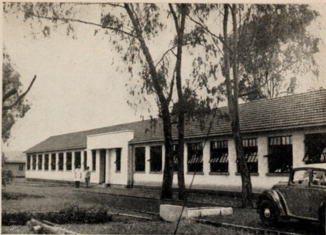
Medical Training School, Nairobi. One of the new buildings
