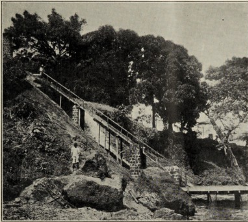
OLD REFUSE CHUTE (NOW DEMOLISHED).
