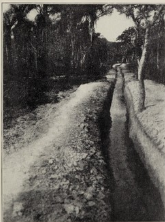
BENDS IN THE STREAM CUT OUT GIVING STRAIGHT RUN FOR WATER.
