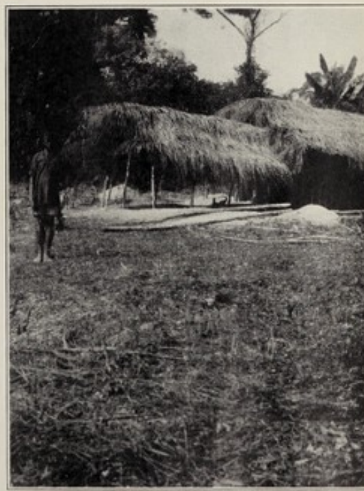
LATRINE COMPLETED; ON RIGHT THE LATRINE PROPER. ON LEFT THE ROOF OVER THE STEPS DOWN TO THE FIREPLACE.
