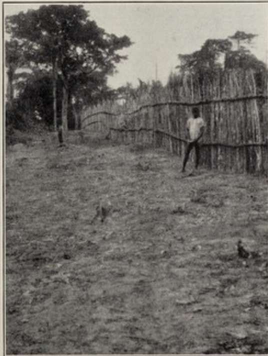
FENCE ERECTED; NOTE HEIGHT COMPARED WITH MAN, AND THE CLEARED AREA OUTSIDE FENCE.
