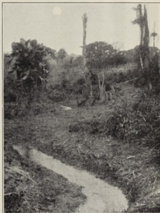
BUSH CLEARED AND STREAM BED CLEANED.
