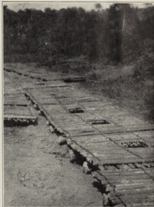
A NUMBER OF SUCH SECTIONS READY FOR PUTTING ON TRENCHES.
