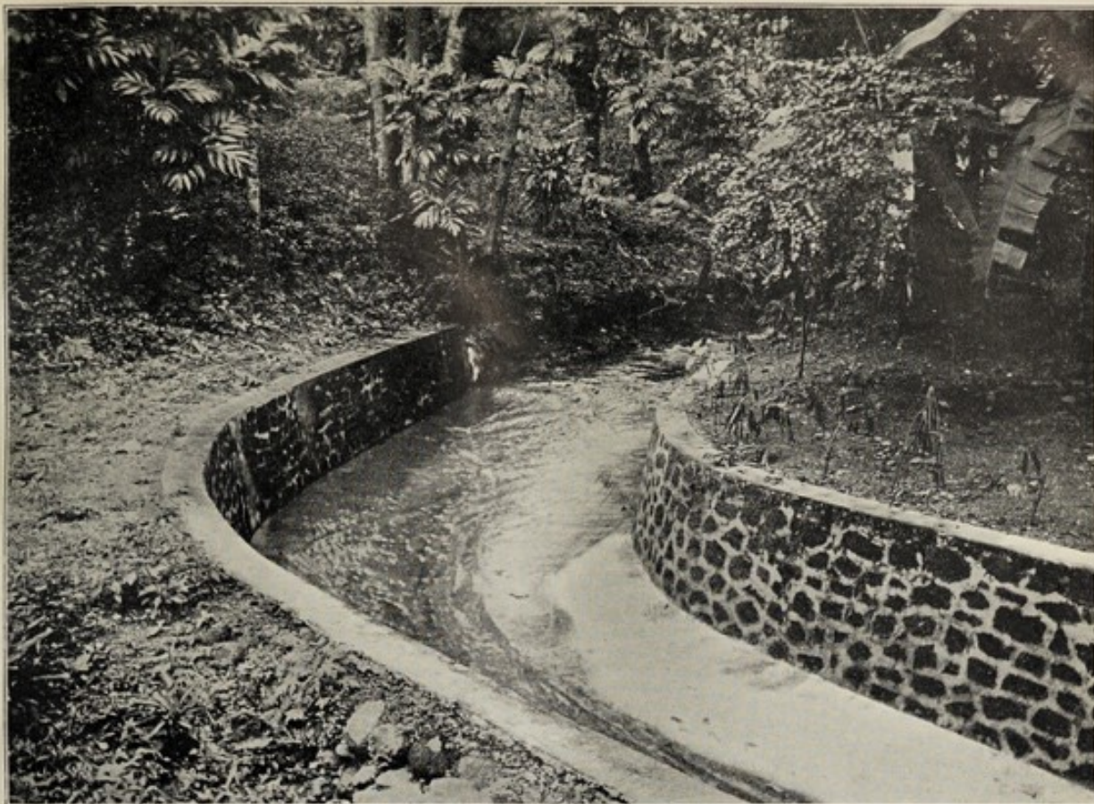
NICOL'S BROOK—SHOWING MODERN CANALISATION.
