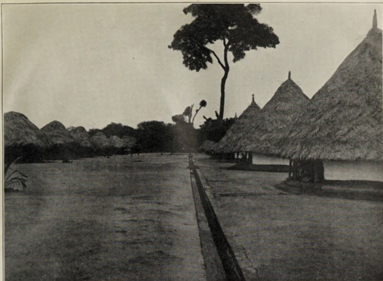
COURT MESSENGERS' LINES, KENNEMA—SHOWING OLD TYPE FLAT-BOTTOMED DRAIN.
