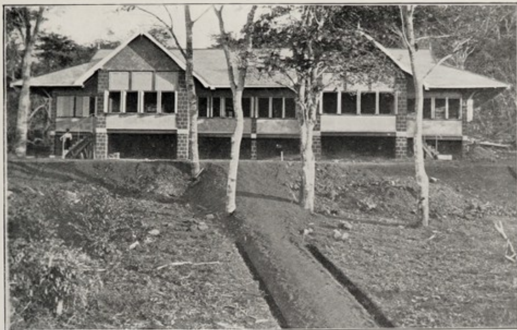
32.—Latest type masonry Double Bungalow with "Eternit" roof; reinforced concrete floor, and Verandah walls; "Steelenite" ceilings (note projection of eaves).
