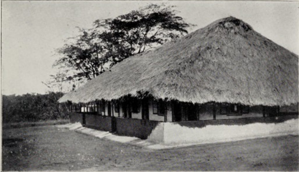
64.—Rest House at Bo (Govt. built). Palm thatch over corrugated iron roof (verandah floor since concreted to throw off water which leaks through thatch and owing to shelter did not dry).
