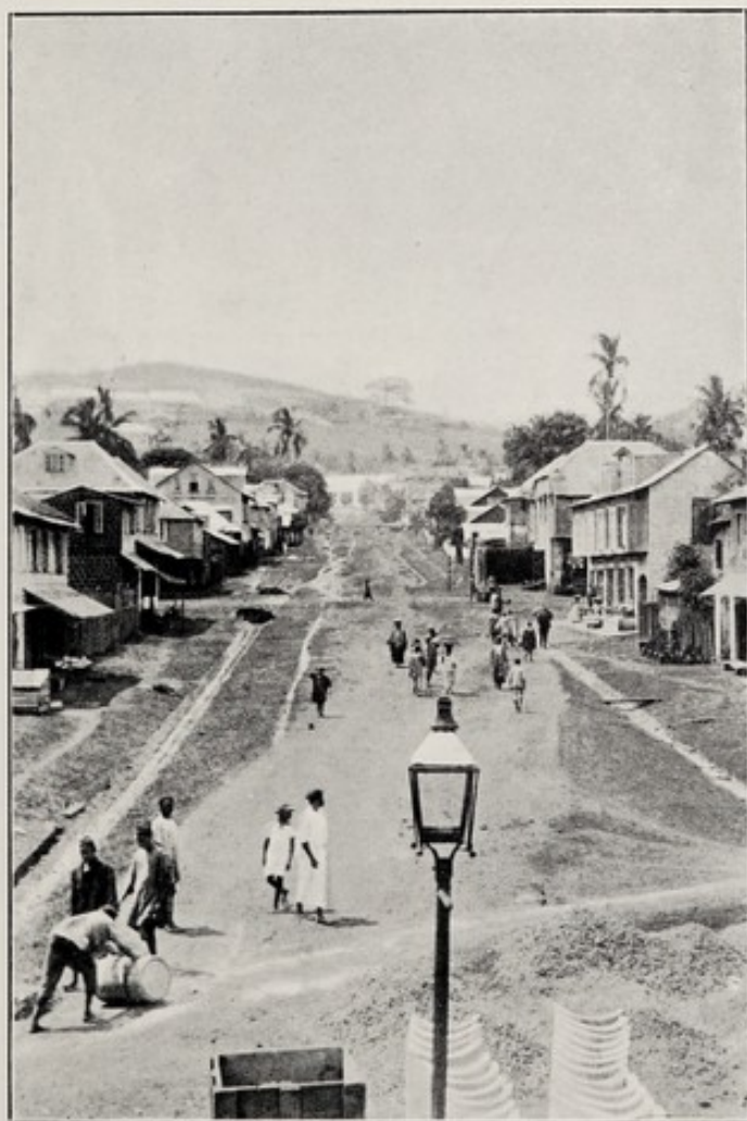
10.—Percival Street; grass-covered street, chiefly at sides, rough masonry drains; concrete drain sections and broken stone in foreground, Tower Hill Barracks in background.
