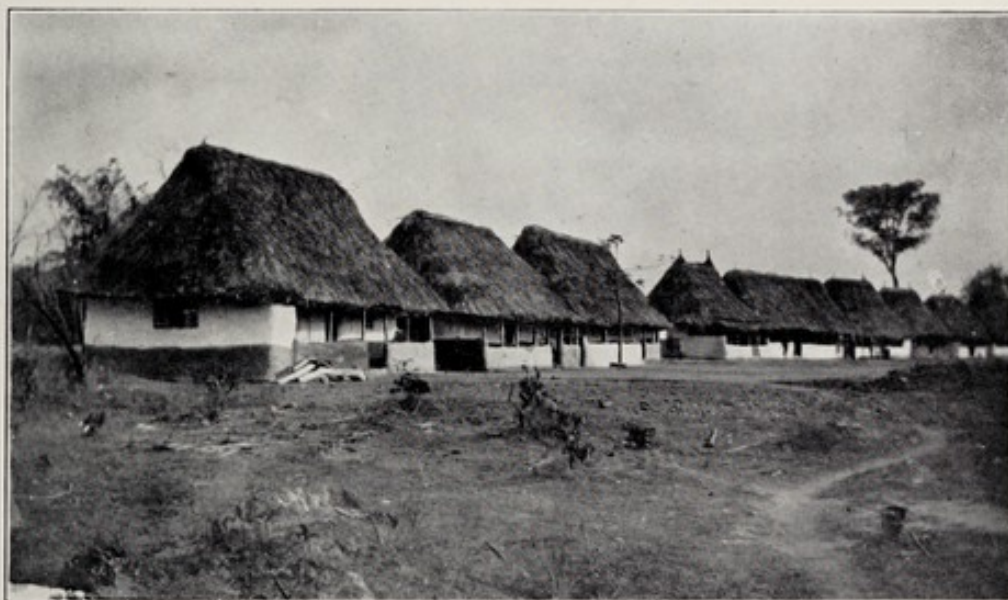
62.—Railway Employees' Houses at Mattru, replacing "shimbeks" similar to those remarked on adversely by Professor Simpson at Bo (Labourers' Qts.).
