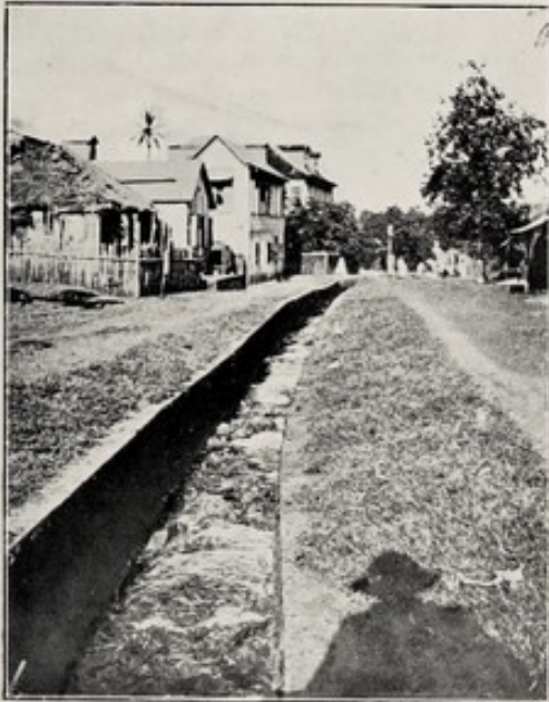
12.—Large old masonry main drain, with flat bottom, perpendicular sides, course in centre of street.
