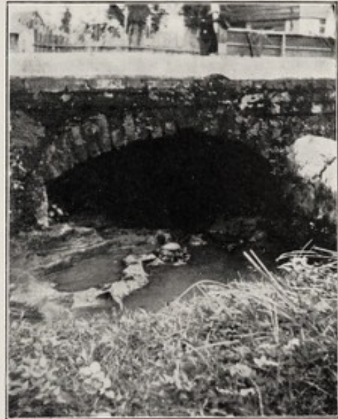
13.—Entrance to large culvert-hole, worn rock, flat bottom (rainy season).
