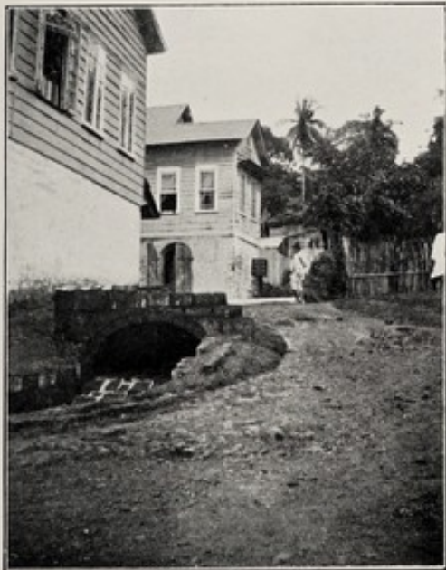
14.—Large masonry culvert and drain.
