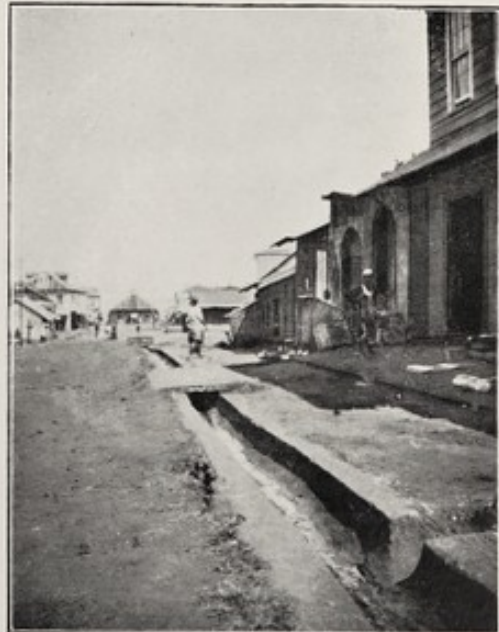
15.—Semi-circular concrete drain (road surface since repaired).
