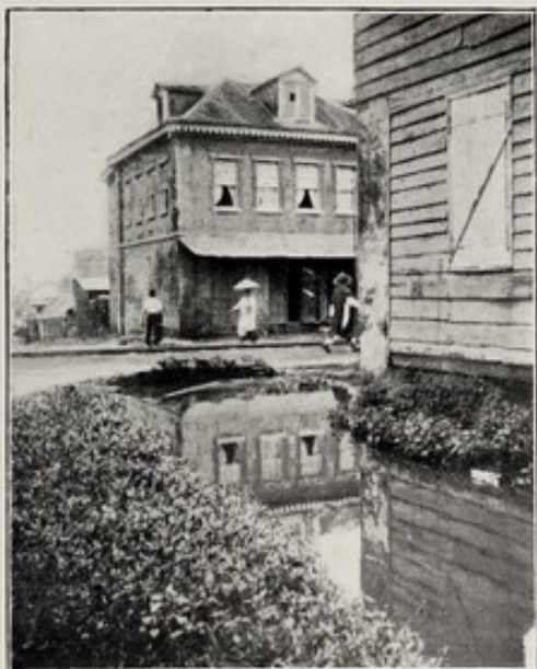
16.—Drain flooded owing to temporary blocking of culvert (rainy season).
