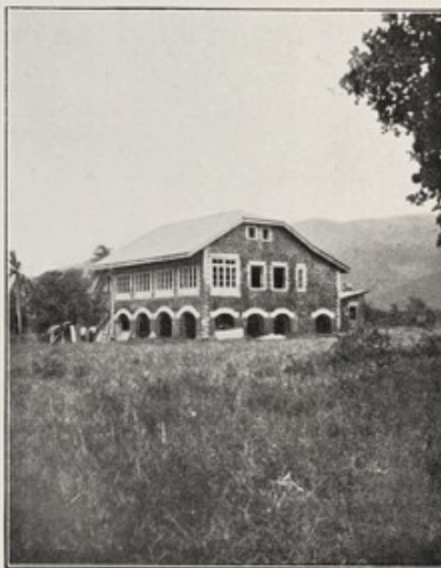
36.—Bungalow at Clinetown (Railway Officials' Quarters).
