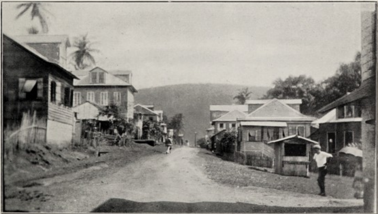
9.—Pademba Road; note grass-covered slopes at Roadside, Wattle Fences, and new type of Refuse Bin.
