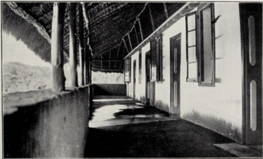
65.—View of verandah of above, shewing arrangement of double roof (thatch).
