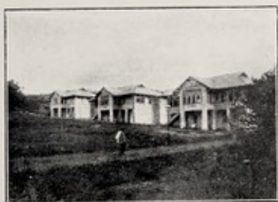
31.—Three new Concrete Bungalows for Officers in Freetown.
