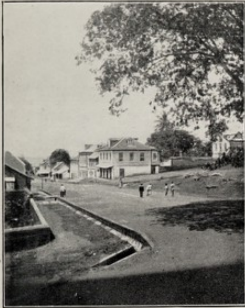
6.—Westmoreland Street, road repaired and new concrete drains laid.
