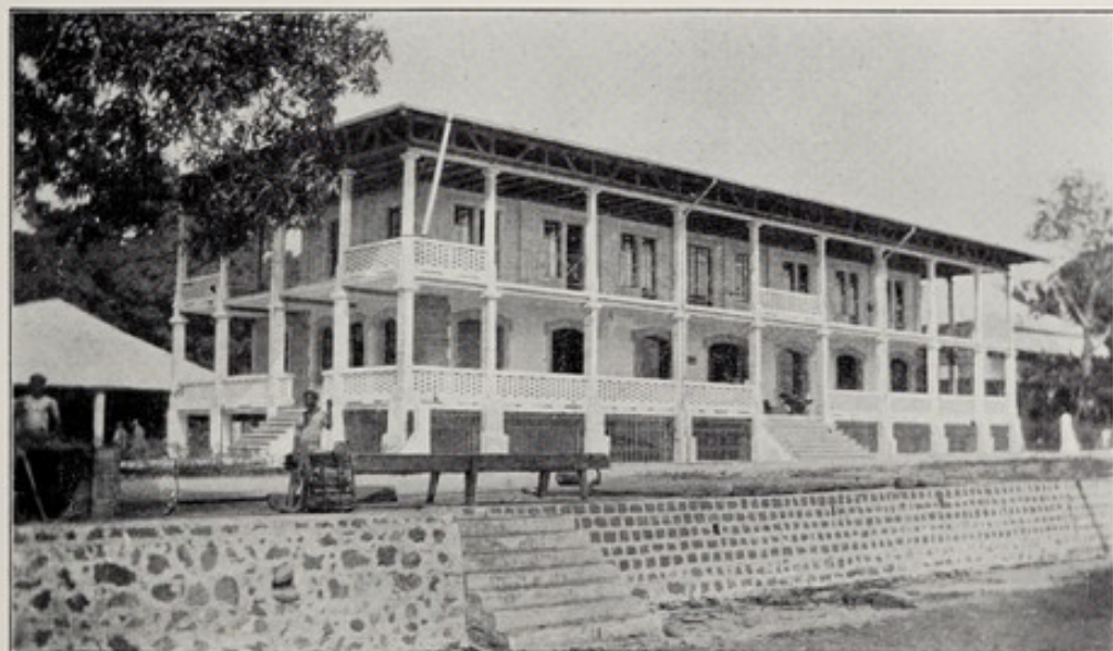
60.—Premises of Swiss trading firm at Bonthe; reinforced concrete.
