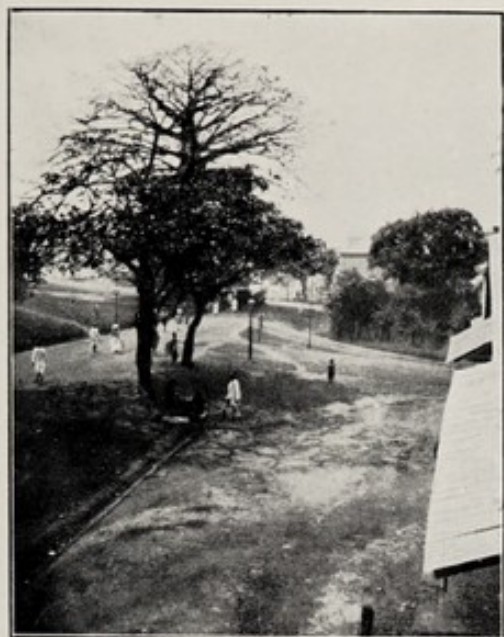
8.—Westmoreland Street, part not yet laid with new concrete drain (note grass-covered slopes).
