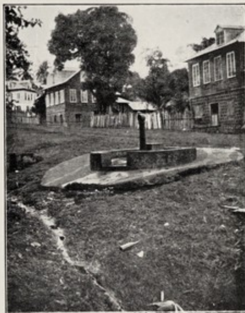
17.—Water supply, street stand-pipe.
