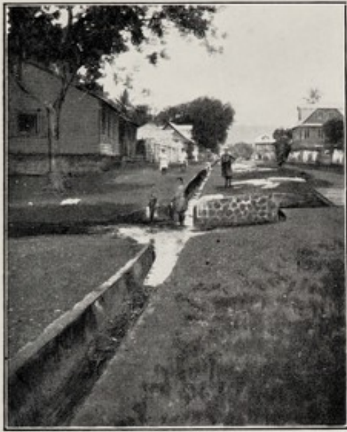
20.—Drain outfall into Sanders' Brook (rainy season).
