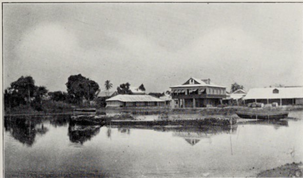
59.—View similar to last, with tide full, taken some months after, and shewing buildings completed, rough turf filling, and further building proceeding as before below high water.
