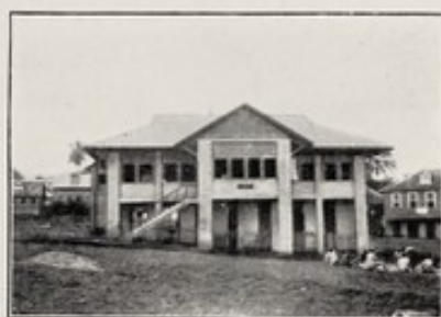
33.—New Bungalow for Comr. of Police in Freetown.
