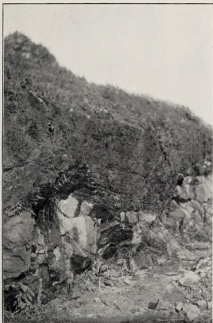
27.—Side of Railway Cutting, subsoil drainage from lower strata of laterite rock, and above Sienite rock underlying.
