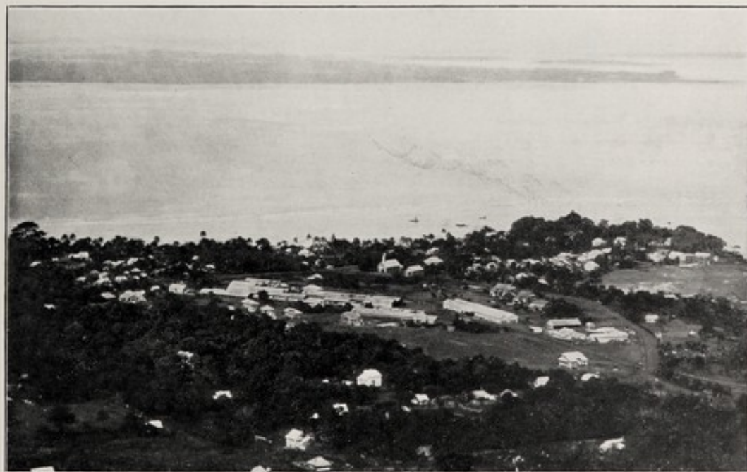
37.—Clinetown Railway Settlement, Works, Stores, Quarters, &c., and Native Town (view from Mount Aureol).
