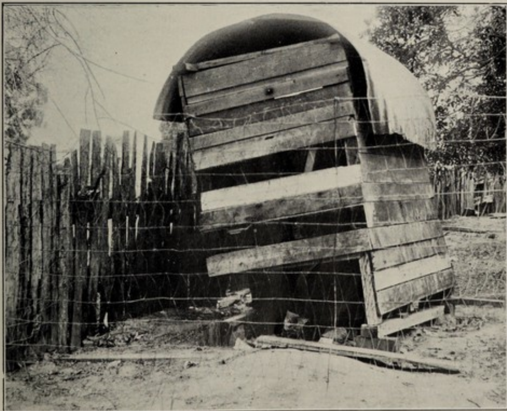
SANITARY CONVENIENCE—Showing how typhoid fever may be transmitted by flies, and which was condemned by the Department.
