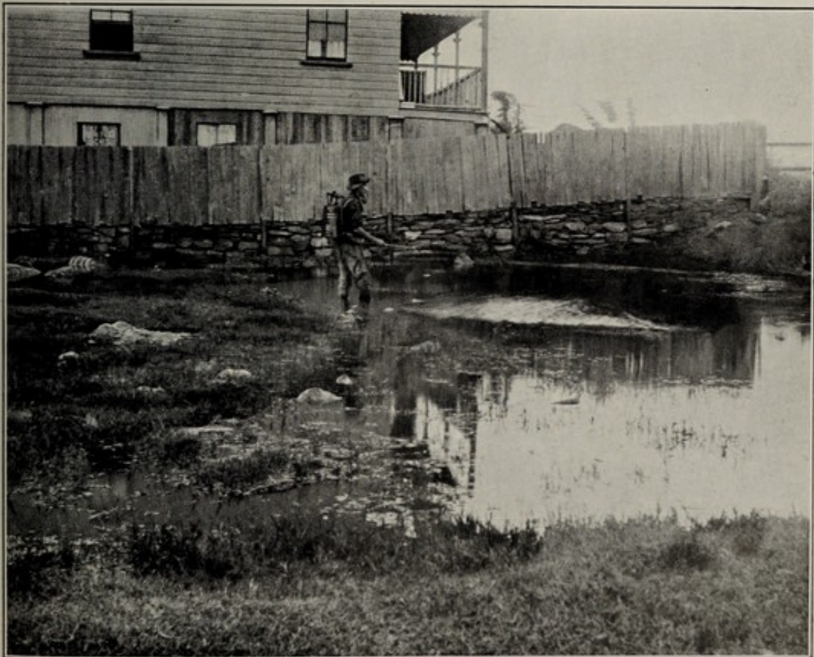
ANOTHER SALT MARSH AT NEW FARM, WHICH HAS ALSO BEEN FILLED IN—Reclamation in each instance has afforded relief to residents in the vicinity.
