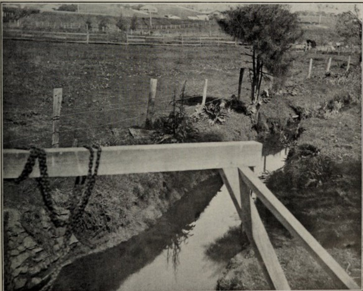
AN EXAMPLE OF A SMALL CREEK, SERVING TO ILLUSTRATE HOW WATERCOURSES BECOME CONTAMINATED BY SEWERS EMPTYING INTO THEM—The invert shown above discharges into this creek at the flood valve, part of which is illustrated in the foreground.
