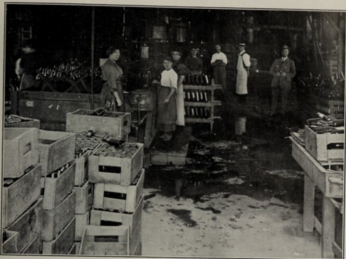
CORDIAL FACTORY AND AERATED WATER WORKS—Poorly lighted and with faulty floor.
