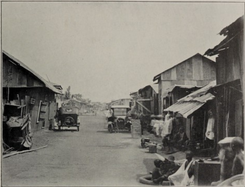
General View of Idoluwo Street, Lagos, a Noted Plague Area, showing Dilapidated and Insanitary Buildings, Galvanized Iron Walls with Inner Bamboo Linings, the spaces between which frequently Harbour Rodents.
