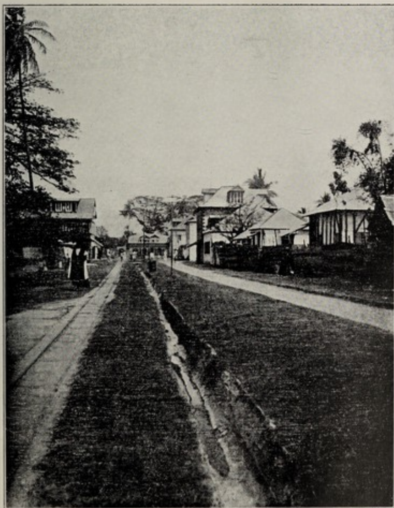
Typical broken and irregular masonry drain. Note collection of water in invert.
