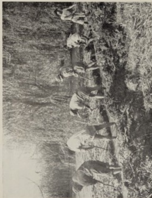
A.—Natives engaged on deepening and regularising south bank of Power Station dam.
