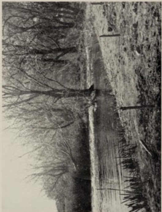
C.—Portion of south bank of Power Station dam, showing a reclaimed clean cut bank with willow cuttings at intervals.
