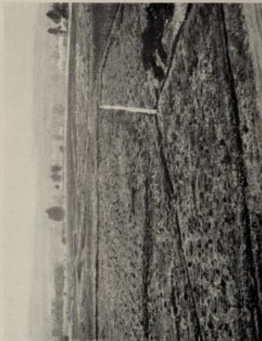
D.—Elimination of seepages by drainage and afforestation. Note fencing and the little mounds where trees have been planted.
