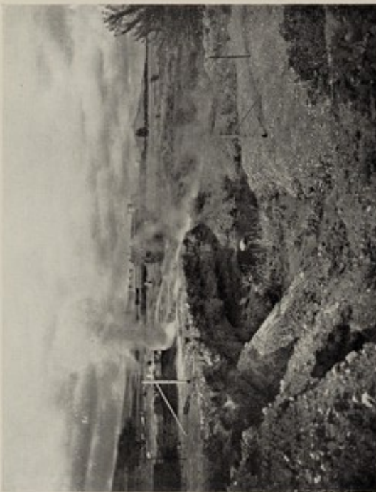
E. Brickfields, Pretoria West. Eradication of a mosquito breeding pool by blasting the sides of the borrowpit with dynamite. Iscor Steelworks in background (17.1.38).
