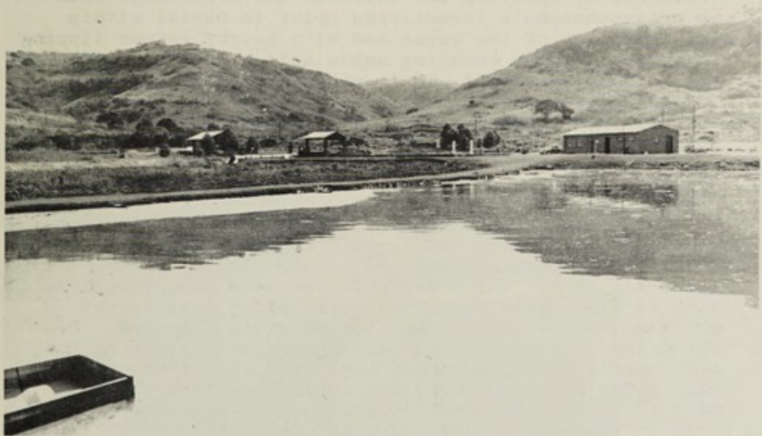
On the left the anaerobic pond 1a with heavy scum formation and growing vegetation, and on the right the anaerobic pond 1b with very slight scum formation.
