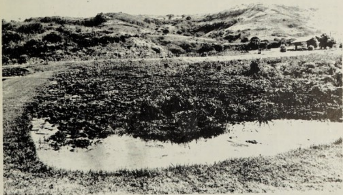
Anaerobic Pond 1a showing heavy scum formation
