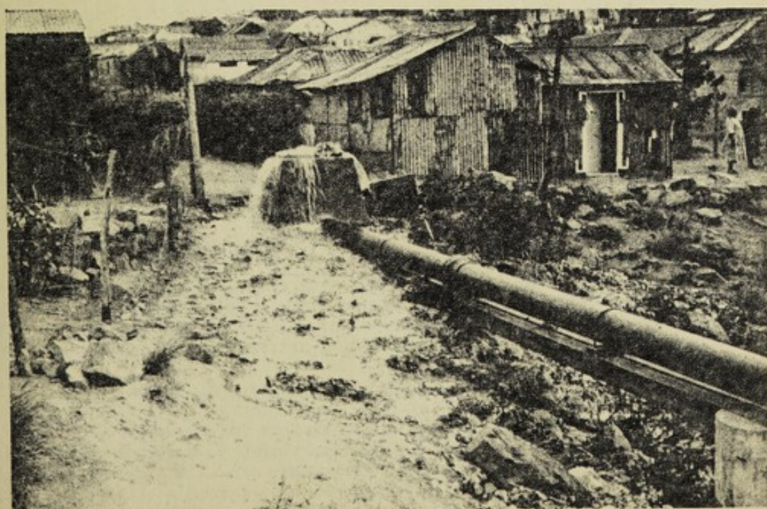
CONSTANTLY RECURRING SEWAGE SURCHARGE DUE TO BLOCK-AGES IN DENSELY POPULATED CATO MANOR AREA
