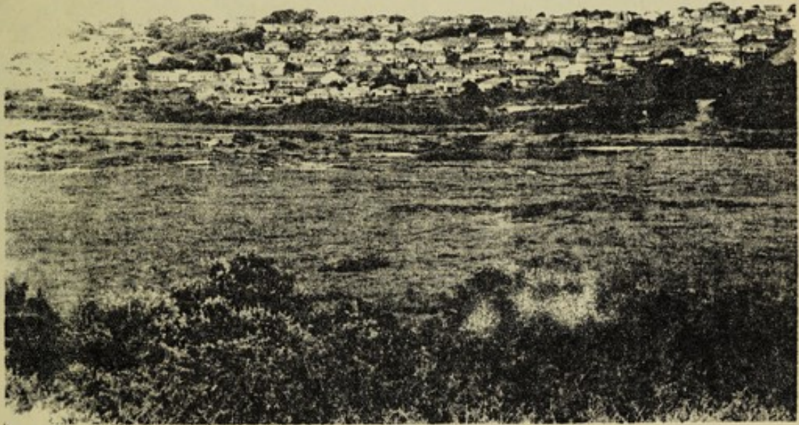
Van Riebeeck Park: Houses from which storm/waste water discharges into swamp.
