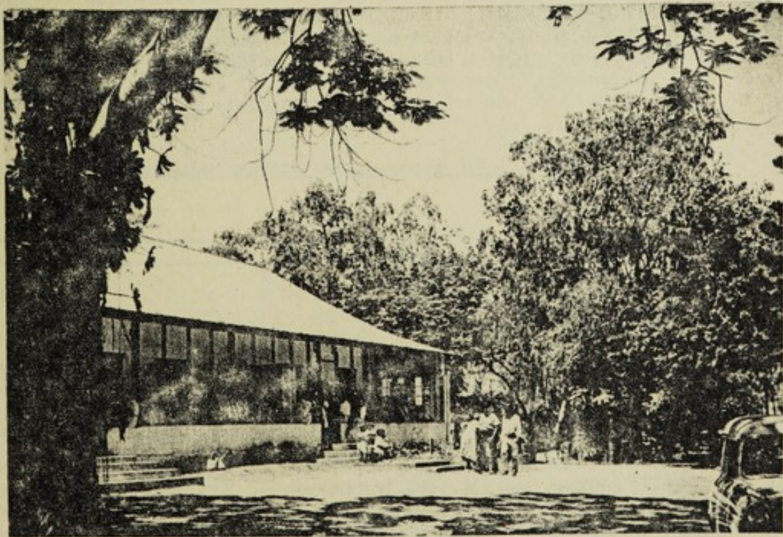
Child Hygiene Clinic serving completed section of new Bantu Township at Kwa Mashu.
