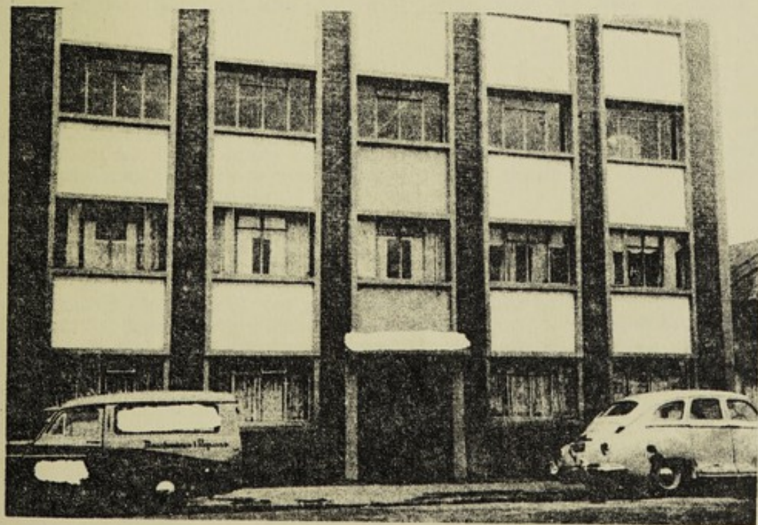
SAME PREMISES AFTER REBUILDING
