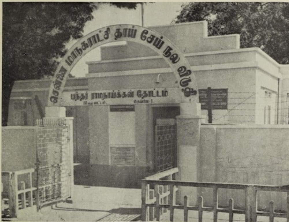
Front view of the newly constructed Child Welfare Centre at Bunder Ramanaicken Garden—12th Dn.
