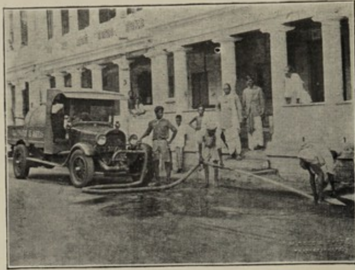
FLUSHING OF THE WATER-TABLES BY MOTOR VAN
