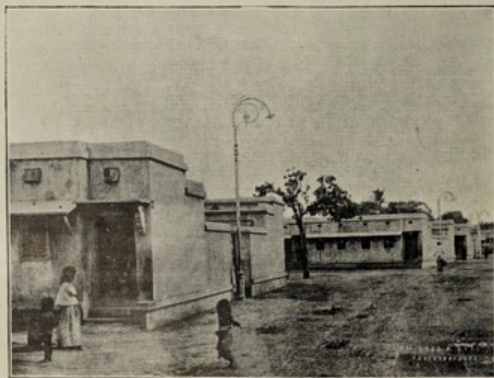
BOGIPALAYAM (AFTER IMPROVEMENTS)
