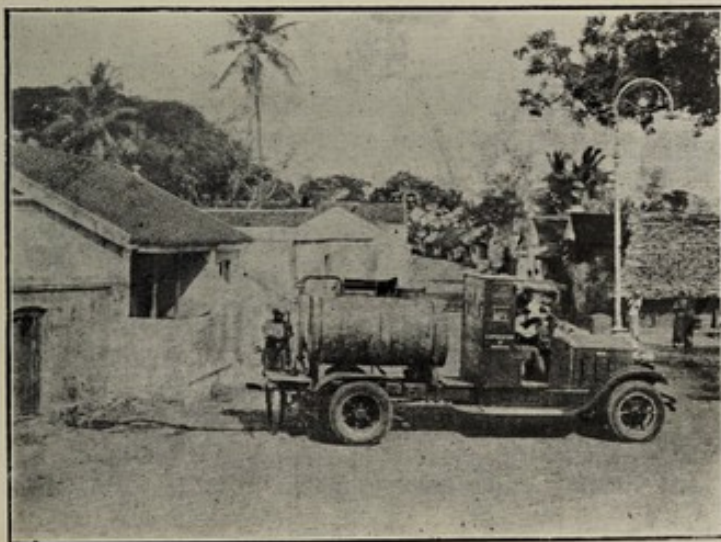
REMOVAL OF CESS POOL CONTENTS BY MOTOR VAN
