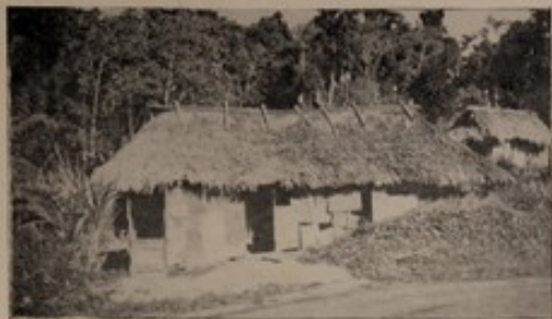
(1) Contractors' "Shanty" for Labourers, Trinidad Leaseholds, Guayaguayare.—April, 1936.
