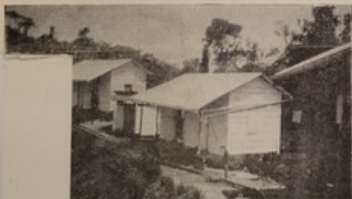
Range of Temporary Barracks, "Abyssinia"—Leaseholds, Guayaguayare—April, 1936.
