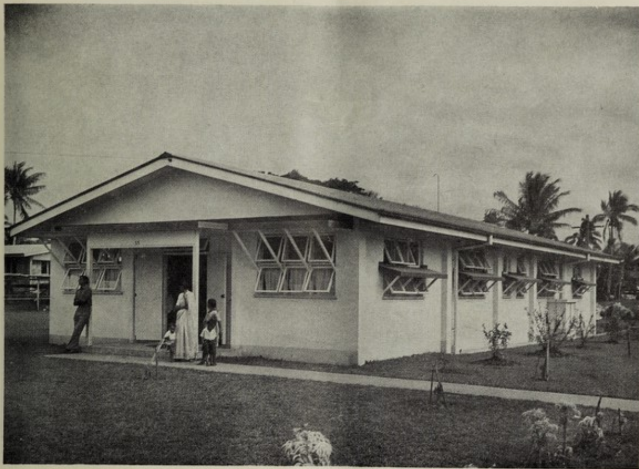
Grade I Rural Health Centre
