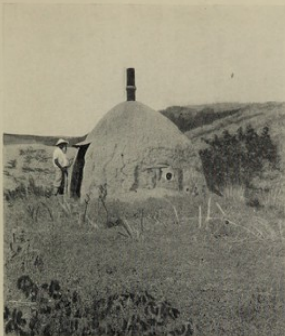
Fig. 4. Old type swish Incinerator; combustion very incomplete; rubbish put in and taken out at same opening; all openings are air inlets or outlets according to direction of wind.
