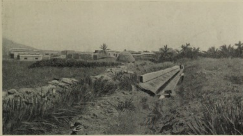
Fig. 10. Lagoon end of new Beulah Lane main drain.
