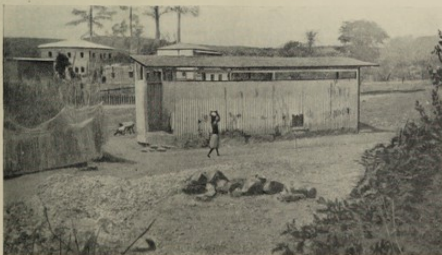
Fig. 6. Old type Latrine; not durable; not drained.
