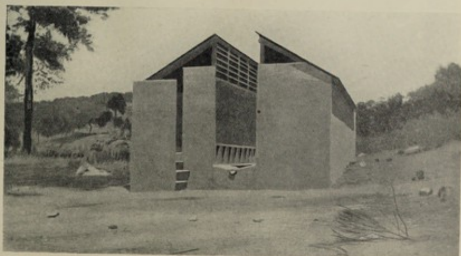
Fig. 9. Concrete squatting pan Latrine. Note passage, drained, between male and female sides. Note openings through which pans removed.
