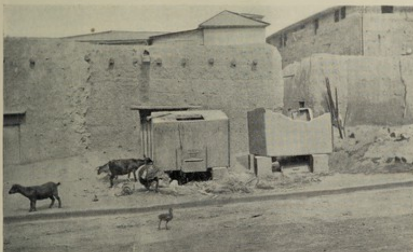
Fig. 5. Old type galvanized iron Dustbins. Goats, fowls, etc., get in and on and scatter the rubbish; not durable. Public will not take trouble to close lid.
