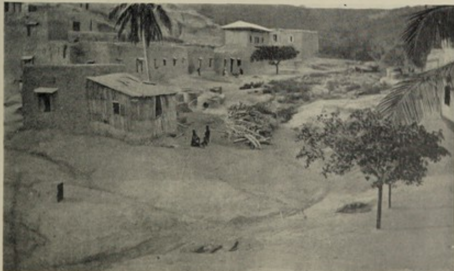
Fig. 12. Water-worn road : Buckman Avenue. No made drains.
