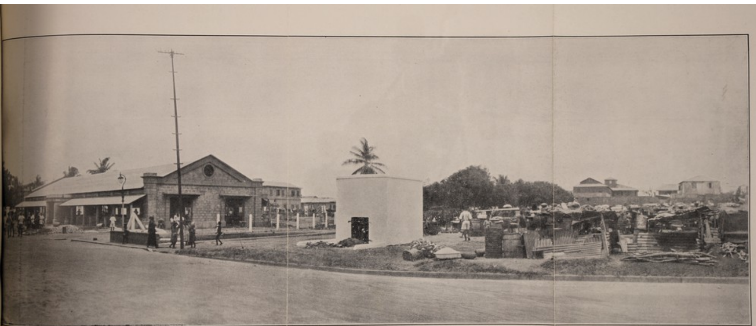
ACCRA. London Market under construction, showing old and new sheds.
