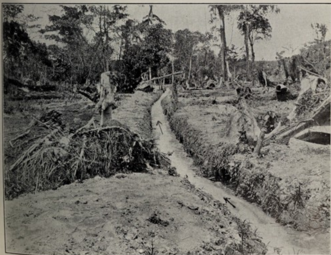
KUMASI, 1929-30. Anti-malarial work. New Asafu Swamp cutting.
