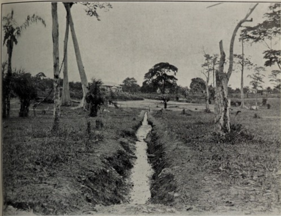
KUMASI, 1929-30. Part of the swamp behind the Residential Area filled in. (Note the proximity of bungalows).
