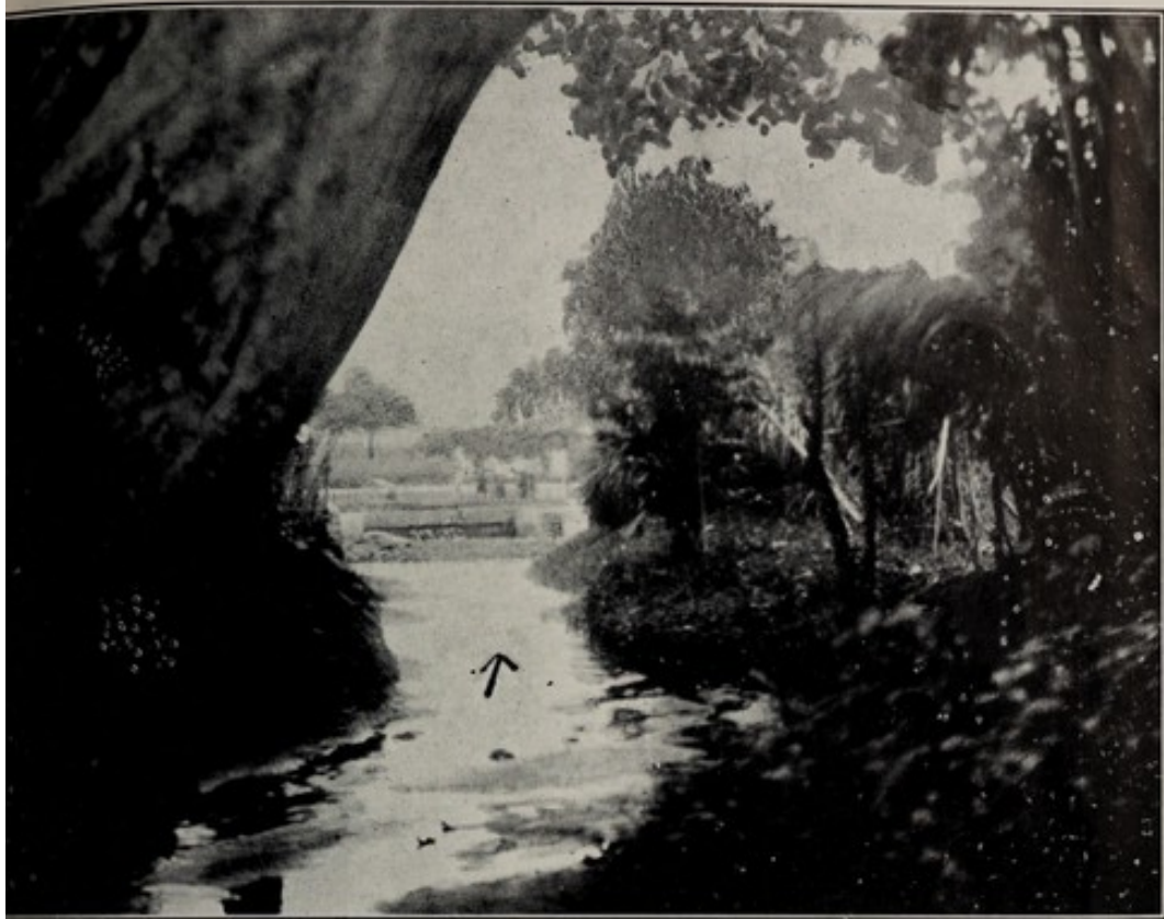
KOFORIDUA. Su Stream at entrance to Catchwater Basins shown below.
