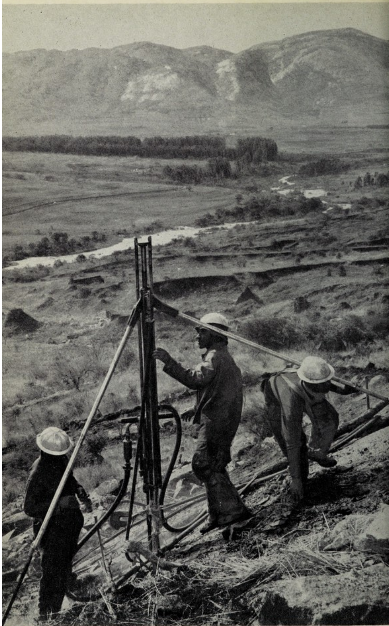
Building the Swaziland Railway. A drilling rig at the site of the tunnels, overlooking the Little Usutu River
