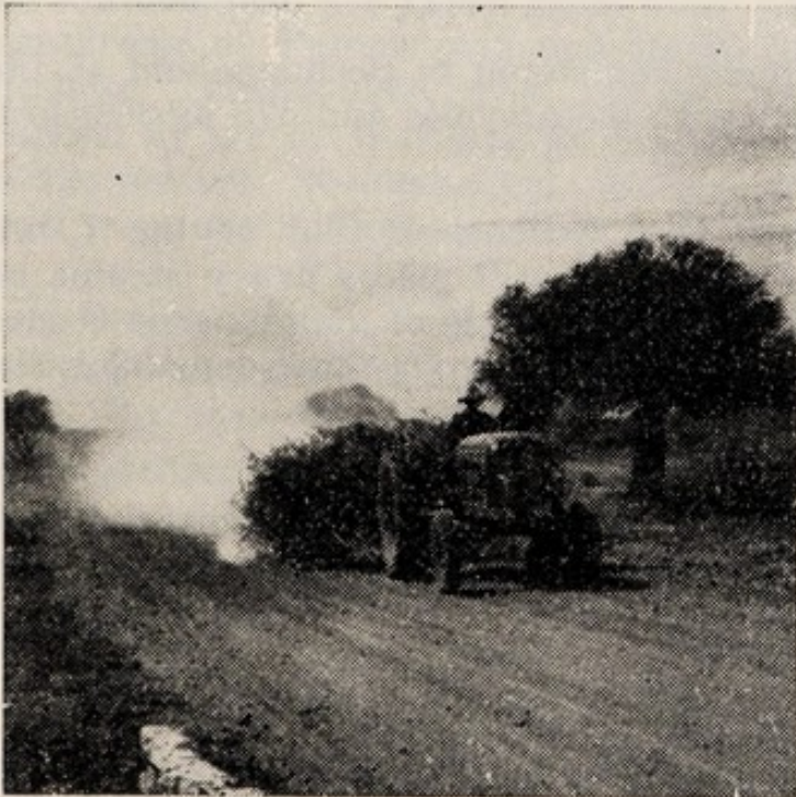
Bush-dragging to prevent formation of corrugations on main road.
