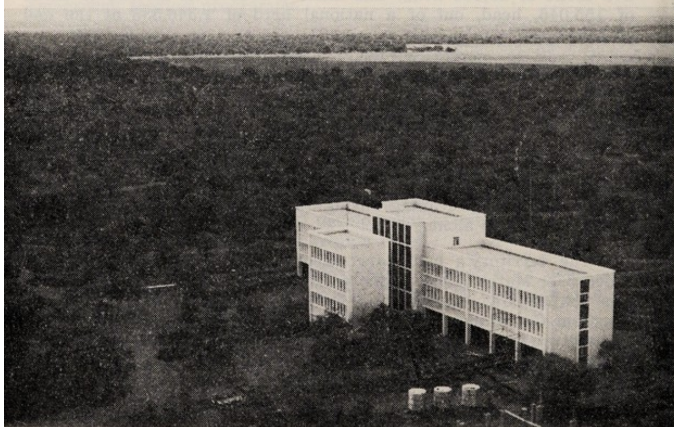
Aerial view of the Prime Minister's Office Block, Gaberones, with foundations of new Ministry of Works and Communications block in foreground.
