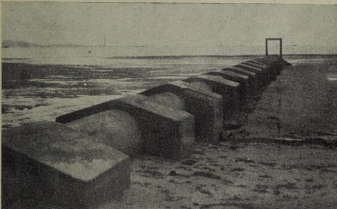
Showing one of the main Anti-Malarial outlets—just repaired (Concrete flume at 12\frac{1}{2} m.s. Changi Road).
