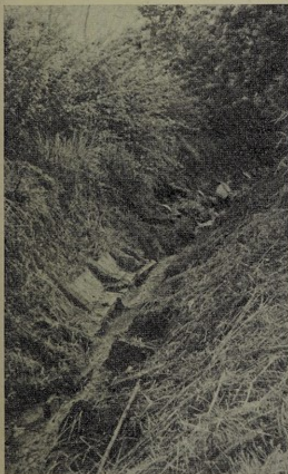
Showing the damage to Anti-Malarial Drain due to lack of maintenance during Japanese occupation. (Municipal Area).
