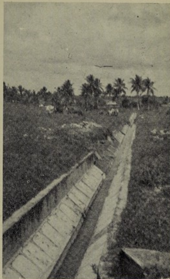
Showing the damage to Anti-Malarial Drain due to lack of maintenance during Japanese occupation. (Serangoon Area).
