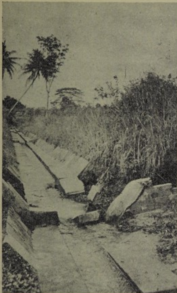
Showing the damage to Anti-Malarial Drain due to lack of maintenance during Japanese occupation. (Changi Area).
