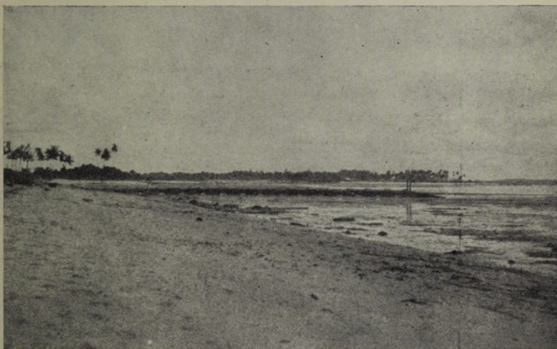
Anti-Malarial main outlet shown—taken beyond sand dome to prevent silting ( 12\frac{1}{2} m.s. Changi Road off Tanah Merah).
