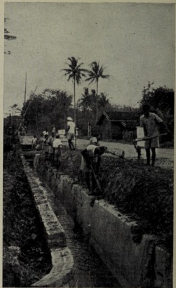
Showing damage to main outlet of Anti-Malarial Drain. Now in process of reconstruction. (Bukit Panjang Area).
