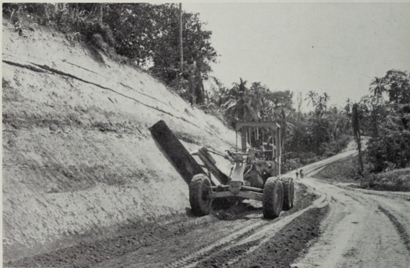
A grader at work on the Gogol Road near Madang.
