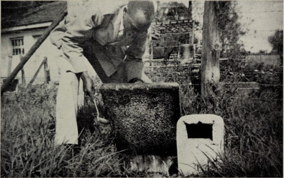
The neglected Septic Tank—cause of much Culicine nuisance
